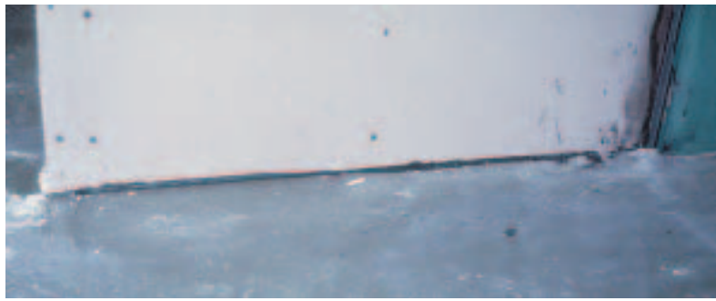
Figure 4. Acoustical sealant under wall plates and around drywall edges seals tiny gaps that might allow transmission of airborne sound.
