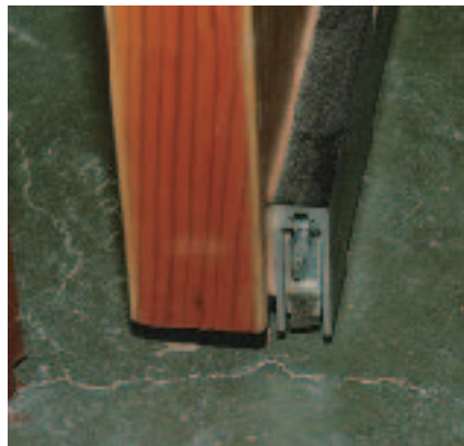
Figure 6. Soft rubber gaskets (left) and an adjustable threshold (right) help close gaps around the shop's doors.
