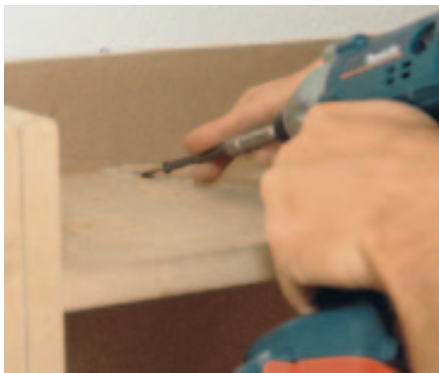
Figure 5. The Mini Kreg Jig comes in handy for installing cabinets and bookcases, and for joints in hard-to-reach places.
