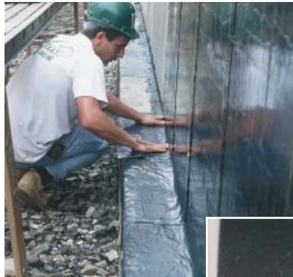
Figure 4. Sheet membranes, like Grace's Bituthene, shown here, apply like peel-and-stick eaves membranes. Inside corners are first coped with proprietary sealants (above left), then the membrane is pressed into place (above right). Most sheet membranes are around 60 mils thick, or about one and a half times as thick as a dime (right).
