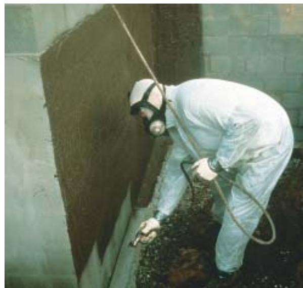
Figure 2. Water-based asphalt emulsion coatings are far less toxic than solvent-based formulations but must be protected from freezing during application.
