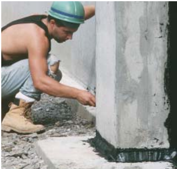
Figure 4. Sheet membranes, like Grace's Bituthene, shown here, apply like peel-and-stick eaves membranes. Inside corners are first coped with proprietary sealants (above left), then the membrane is pressed into place (above right). Most sheet membranes are around 60 mils thick, or about one and a half times as thick as a dime (right).
