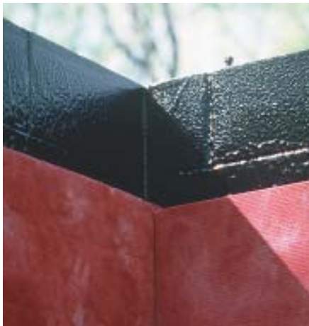
Figure 5. Protective insulation and drainage boards are often incorporated into foundation waterproofing systems. Shown here are Koch's Tuff-N-Dri (above), which includes a foundation board from Owens Corning; and HouseGuard's Tru-Dry (right), which uses a Dow Styrofoam insulation and drainage board.
