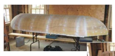
The bendable plywood skin of the "hull" draws its support from curved plywood ribs. Tarpaper templates were used to plot the vertical joints between the straight central section and the tapered ends.
