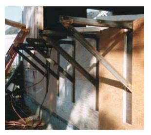
Welded angle-iron brackets attached to the framing provide structural support for the bay window. Access holes were later cut into the sheathing between brackets to permit screwing the nonstructural apron to the brackets from within.
