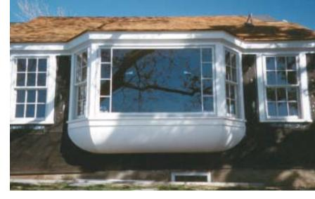
The epoxy-bonded curved plywood apron beneath this waterfront bay window was designed to mirror the forms of the boat hulls moored just beyond the lawn.
