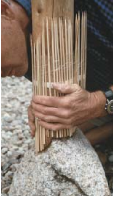
Figure 2. The tip of each skewer, affixed on bands of double-stick tape, defines the contour line of the stone at the perimeter of the post pattern. The author then used chalk to transfer high points from the stone and hollowed the pattern's end accordingly.
