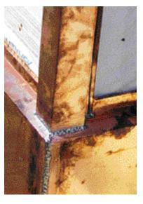
The 16-ounce copper corner trim and water table were formed on a bending brake and soldered on site. A right-angle bend at the upper edge of the water table acts as a "starter course" to hold the bottom of the first course of slate clear of the sheathing. Each slate is fastened to the <sup>5</sup>/8-inch plywood sheathing with two 1<sup>1</sup>/2-inch copper nails.
