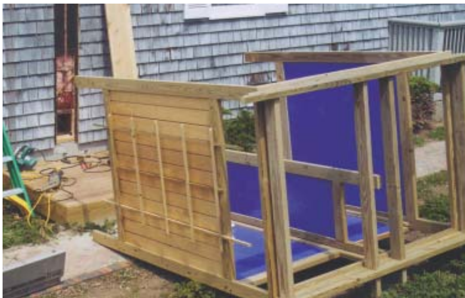
Figure 2. The exterior T1-11 plywood siding has one "good" face, left to weather on the public side. The rough backing veneer within the enclosure is painted with gloss-finish latex trim paint.
