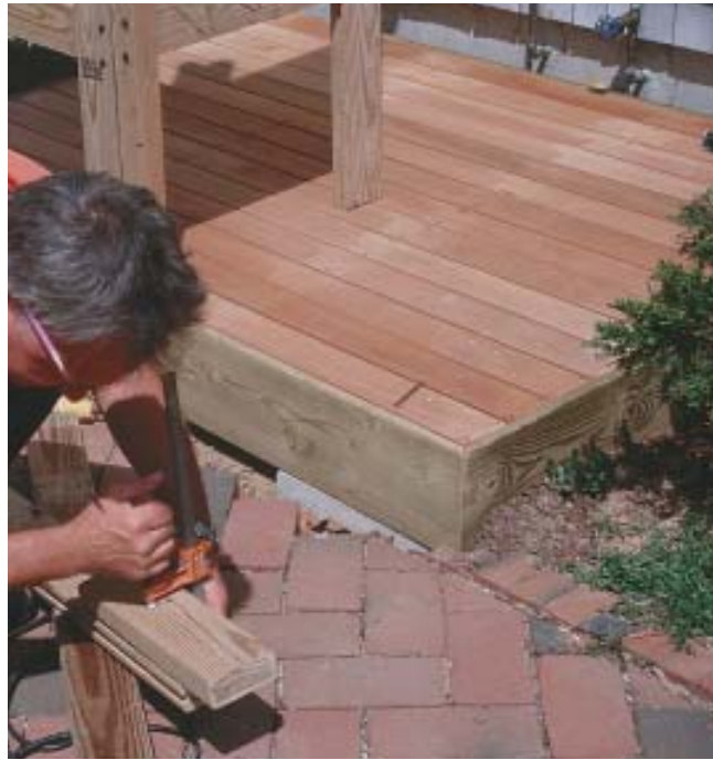
Figure 3. A raised wood platform prevents muddy feet. A rabbetted and mitered rim joist and recessed framing make a built-in border around the decking edge. Stainless-steel decking screws eliminate potentially painful nail pops.
