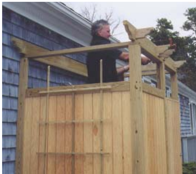
Figure 4. Overhead framing braces panels and maintains a fixed door opening (left). A decorative pergola can support semiconcealed piping and a rain-shower head (below).
