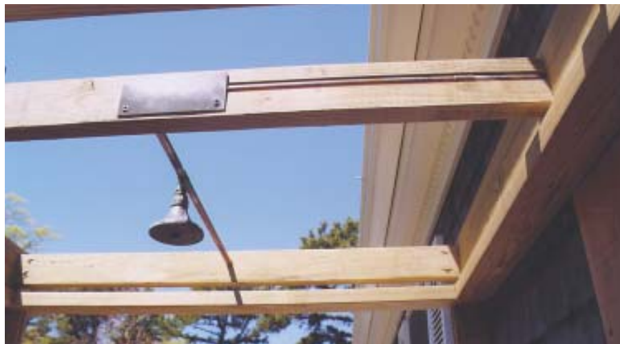
Figure 4. Overhead framing braces panels and maintains a fixed door opening (left). A decorative pergola can support semiconcealed piping and a rain-shower head (below).
