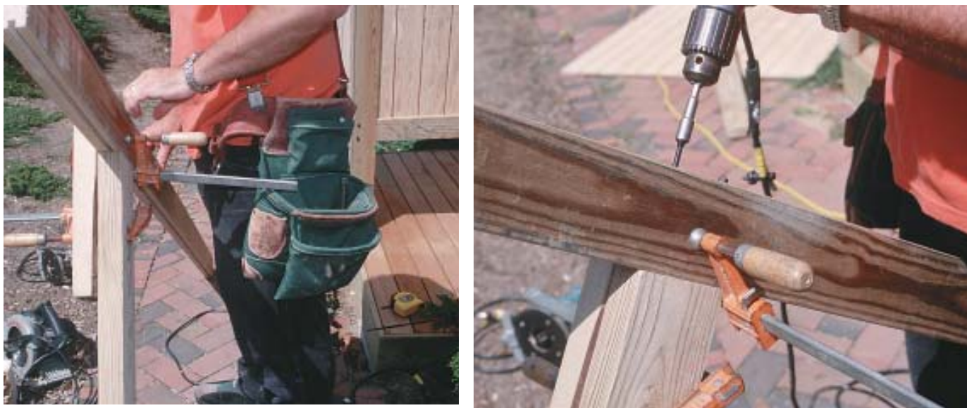
Figure 1. The author's frame-and-panel method simplifies enclosure assembly. Edge-dadoed frame members are butt-joined on the flat, held in alignment with cauls and clamps (left), and lag-bolted together (right).
