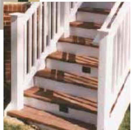
Figure 3. Built-in lighting adds after-dark atmosphere and improves safety. Low-voltage sconces are installed in the deck posts (left), and step lights in the stair risers illuminate the treads (below).
