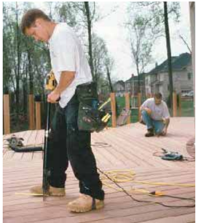
Figure 8. The decking is fastened with trim-head screws, which are buried slightly below the surface of the composite decking. Each screw creates a small “mushroom” that is hammered flat to conceal the screw head.
