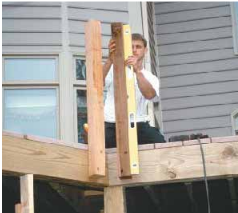
Figure 10. A temporary “hanger nail” driven into a pre-cut post at the level of the deck surface provides temporary support while the post is tack-nailed in place before bolting (below). To provide a simpler, stronger installation, posts are paired at either side of angle transitions and corners. The 4-inch gap between posts corresponds to the standard baluster spacing (left).
