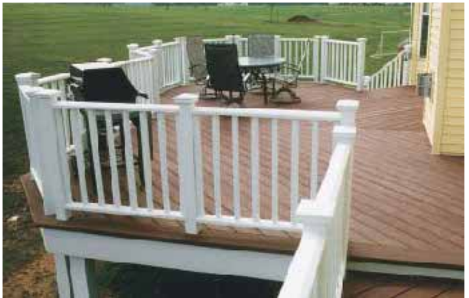
Figure 2. The author's base-priced deck uses a square-baluster-and-rail system, but a broad range of additional styles are available for a variable upcharge, which is calculated by the linear foot. The ornate Chippendale railing (below) is a premium-priced option, while the Madison Colonial (right) is a more modest upgrade.
