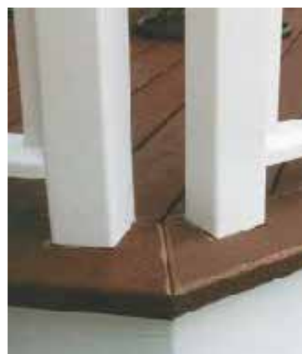
Figure 1. In an optional upgrade to the standard bolt-on post system, the deck boards are cut flush with the girder, and 2x4 cleats are nailed between the posts (top right). A 2x10 finish band joist is then fastened to the faces of the posts, followed by a 2x8 laid flat and notched around the posts (above). The embedded posts have a strong visual connection with the deck, while the overhang at the band joist creates an attractive shadow line (right).
