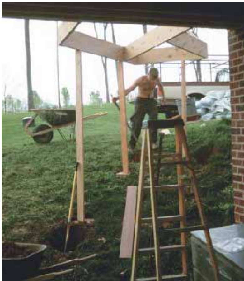
Figure 6. The basic frame of the deck is assembled on temporary posts placed where they won't interfere with the permanent posts (above). The site for each footing is determined with a plumb bob, and the holes are dug by hand (above right). Once the concrete piers have been finished flush with the grade and drilled to accept an expansion bolt, the posts are fastened to post anchors with a palm nailer (right).
