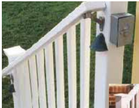
Figure 3. Built-in lighting adds after-dark atmosphere and improves safety. Low-voltage sconces are installed in the deck posts (left), and step lights in the stair risers illuminate the treads (below).
