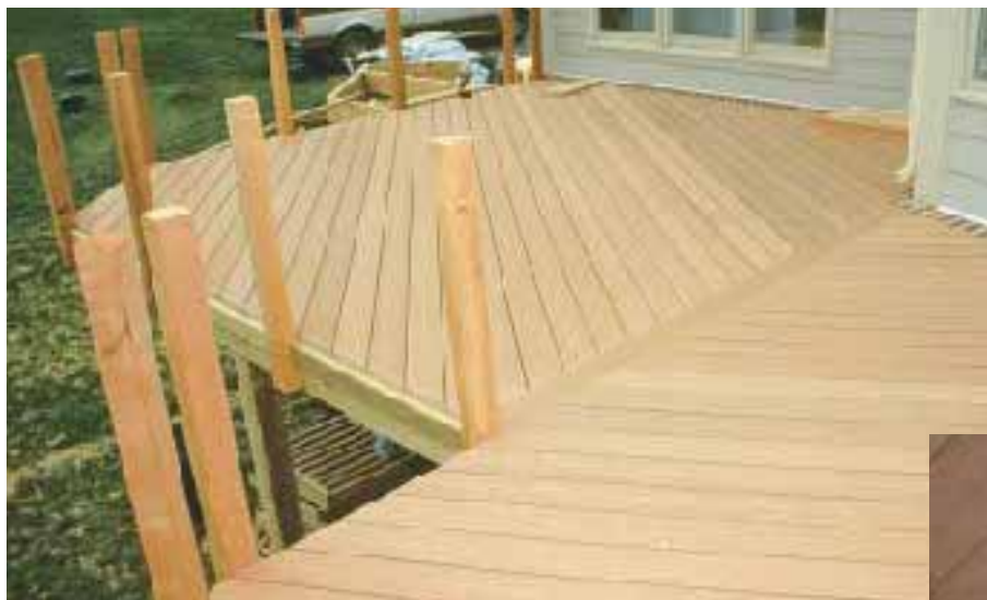
Figure 7. Running the deck boards diagonally eliminates unsightly butt joints. The layout is planned so that no individual board will be longer than 20 feet (above). Joists are spaced on 1-foot centers to provide a stiff surface underfoot. Where adjacent diagonal runs meet, an inlet strip, fastened to blocking between joists (right), provides a pleasing transition.
