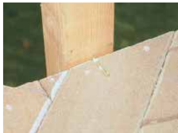
Figure 10. A temporary “hanger nail” driven into a pre-cut post at the level of the deck surface provides temporary support while the post is tack-nailed in place before bolting (below). To provide a simpler, stronger installation, posts are paired at either side of angle transitions and corners. The 4-inch gap between posts corresponds to the standard baluster spacing (left).
