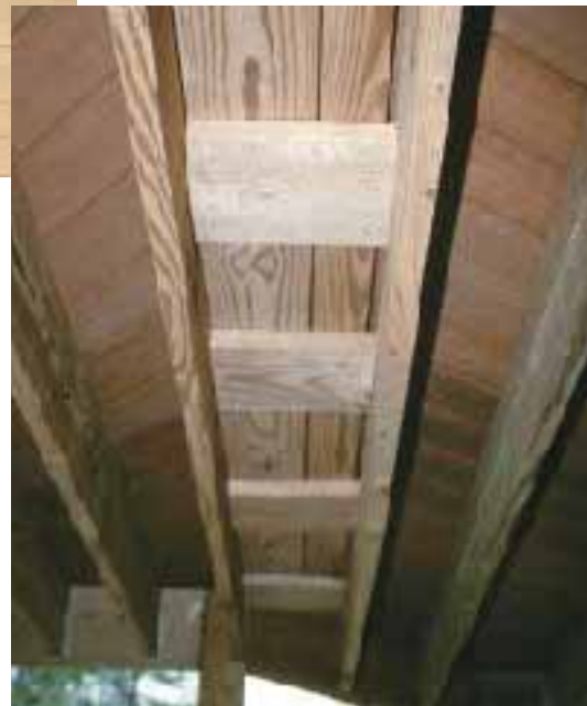
Figure 7. Running the deck boards diagonally eliminates unsightly butt joints. The layout is planned so that no individual board will be longer than 20 feet (above). Joists are spaced on 1-foot centers to provide a stiff surface underfoot. Where adjacent diagonal runs meet, an inlet strip, fastened to blocking between joists (right), provides a pleasing transition.
