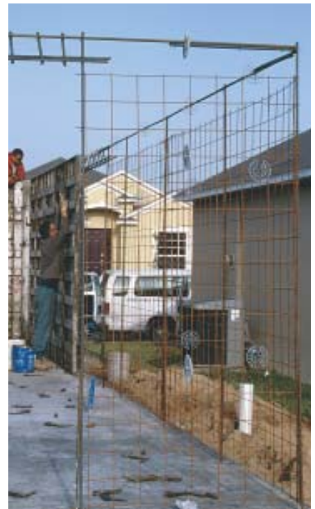
Figure 3. Six-inch-square welded wire mesh is centered between forms with the aid of plastic spacers placed on 4-foot centers. Mesh sheets are started at the building corners, and runs overlap 12 inches.
