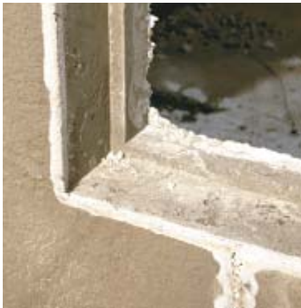
Figure 6. Windows are installed from the outside of the wall and are pressed into a continuous bead of silicone sealant against a \frac{7}{8} -inch offset lip cast in the opening. The installation tolerance is tight, typically only about \frac{1}{4} inch over the unit dimension, to minimize air infiltration around the window.
