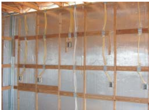
Figure 9. Foil-faced \frac{3}{4} -inch-thick polyisocyanurate foam board is nailed to the interior wall surface and strapped on 2-foot centers with vertical 1x3 furring strips to receive the drywall. The furring and electrical boxes are nailed to the wall with PAFs.
