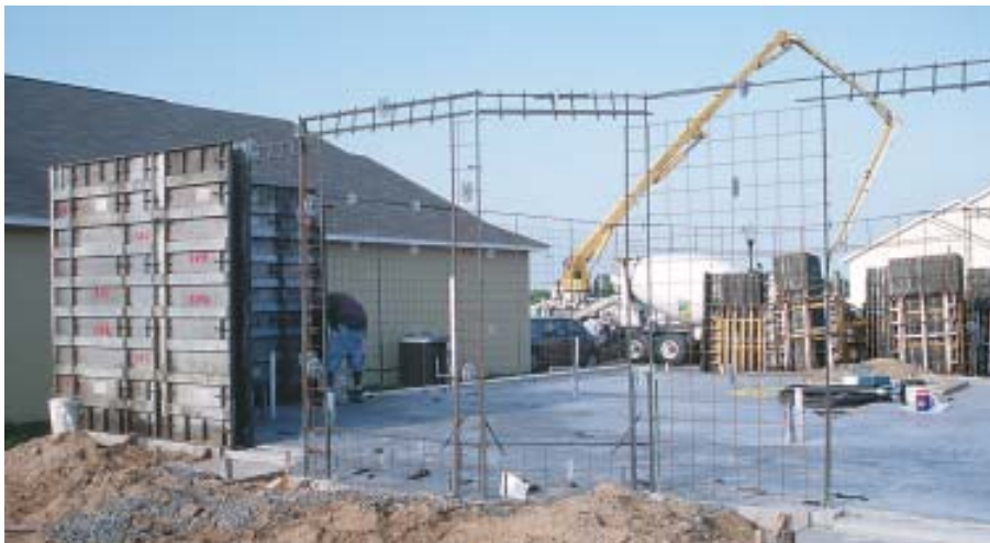
Figure 1. The author installs cast-in-place walls on the thickened edge of a slab-on-grade building platform. No. 5 rebar “up-rods” are wet-set into the slab and, once cured, wire-tied to the wall reinforcement.
