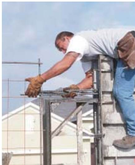
Figure 2. The typical concrete window header is 16 inches deep and is reinforced according to the particular design load.
