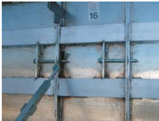
Figure 5. Attached captive pins are affixed to the face of each aluminum form on 12-inch centers. The pins pass through flat steel snap-ties before engaging the next form in line. Adjustable guide-ties enable proprietary window bucks to hang on the pins, automatically leveling the bucks in the forms.
