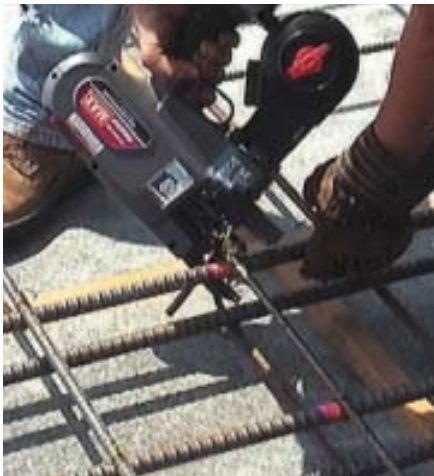
Figure 4. A mechanical rebar tie gun can make a secure connection in less than a second.
