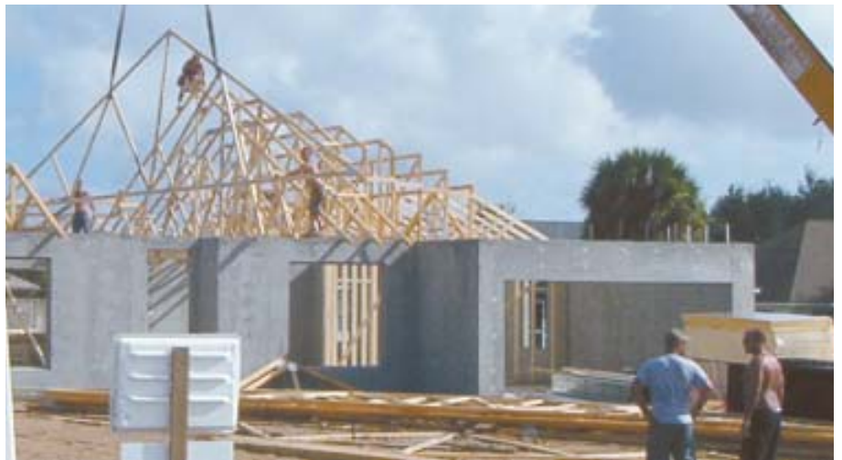
Figure 7. Truss anchors must be accurately placed in the wet concrete, within 1/8 inch of the truss location to perform as designed. The anchor is embedded 4 to 6 inches into the concrete and wrapped over the top of the truss, then nailed. The anchors are rated to resist 120 mph wind uplift.
