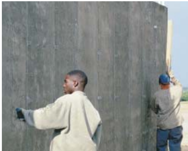
Figure 8. Wall ties snap on impact; those out of easy hammer reach fall to a length of 2x4. The forming crew leaves the slab broom-clean for the framers.
