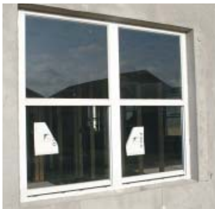
Figure 6. Windows are installed from the outside of the wall and are pressed into a continuous bead of silicone sealant against a \frac{7}{8} -inch offset lip cast in the opening. The installation tolerance is tight, typically only about \frac{1}{4} inch over the unit dimension, to minimize air infiltration around the window.
