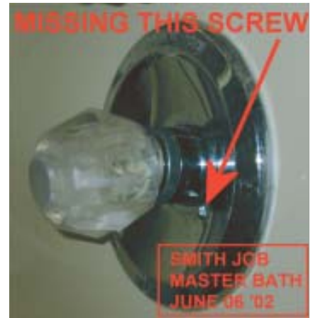
Figure 3. Missing or damaged components can be easily documented using a digital camera and an image-editing program that can add captions and markup.
