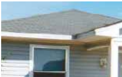
Figure 1. Florida Solar Energy Center researchers compared the air-conditioning power use of seven identically built houses with different roof coverings. Reflective roofing dramatically reduced total power use (bottom chart) and had an even greater effect on peak A/C power demand (middle chart). Insulating the roof deck and sealing the attic, without using a reflective roof, cut total energy use somewhat but did not reduce peak cooling loads noticeably.
