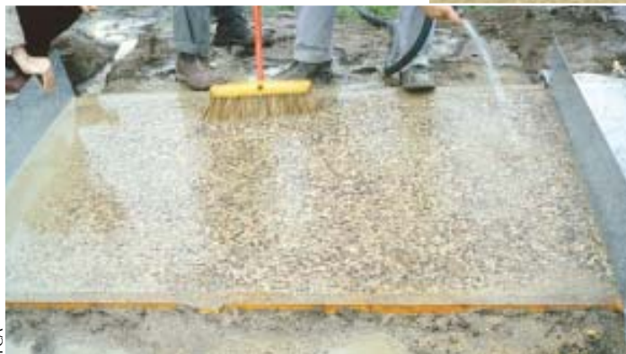
PCA An exposed aggregate finish is the product of a hose and a stiff broom.
