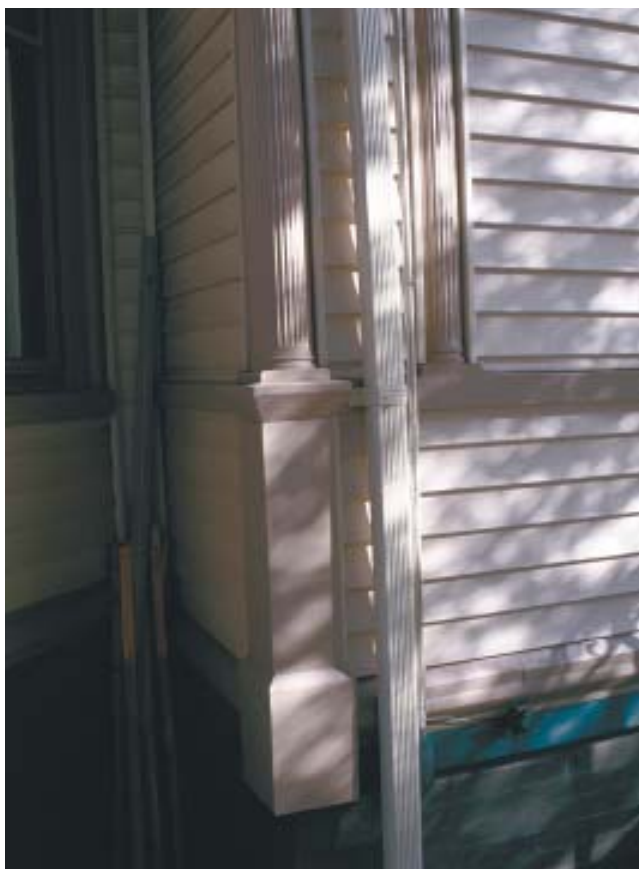
Figure 5. Like the rest of the wood trim on this period structure, these wood columns were repainted before the siding was applied. The column base and adjacent horizontal trim are aluminum.
