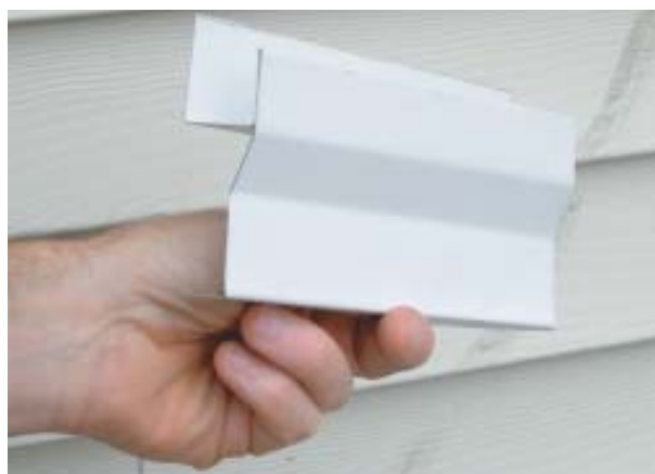
Figure 2. The vertical leg of this site-bent window casing stock is designed to be fastened to the wall with stainless-steel nails that are concealed by the siding. Mitered corners where the side and head casing meet are secured with a single stainless-steel face nail. The lower horizontal leg is dimensioned to wrap around the window casing and be caulked in place (above). The base of the side casing is caulked to the aluminum-clad sill to provide a clean-looking “J-less” window surround (left).
