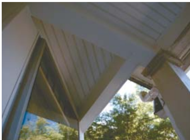
Figure 3. Beaded vinyl soffit has been applied to this porch ceiling (left); the headers are clad with prepainted aluminum coil stock. The tapered square columns will be refinished with paint. Vinyl’s natural flexibility is useful for many trim applications. This curved soffit closely resembles the original version, which was made from tongue-and-groove boards (right).
