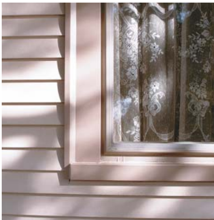
Figure 2. The vertical leg of this site-bent window casing stock is designed to be fastened to the wall with stainless-steel nails that are concealed by the siding. Mitered corners where the side and head casing meet are secured with a single stainless-steel face nail. The lower horizontal leg is dimensioned to wrap around the window casing and be caulked in place (above). The base of the side casing is caulked to the aluminum-clad sill to provide a clean-looking “J-less” window surround (left).
