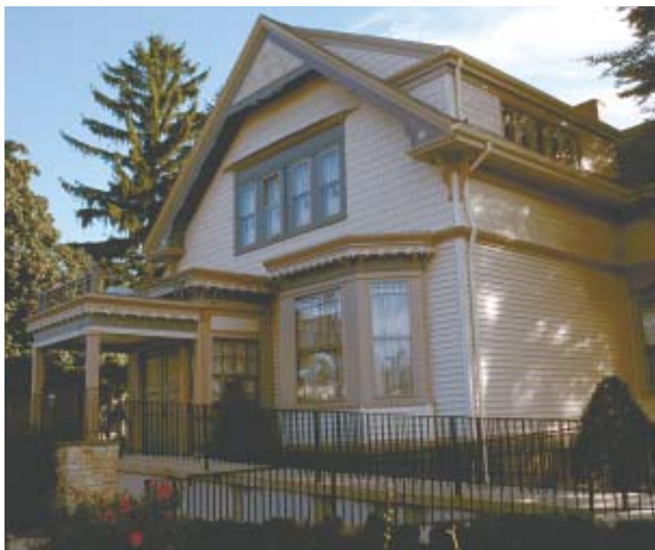
Figure 4. A well-thought-out combination of polypropylene shingles, vinyl siding, site-bent aluminum trim, and original wood trim gives little indication that this older house is not sided entirely with wood (left). The eaves brackets and carved fascia with its ornamental “canoes” are original. Soffits are vinyl, while the frieze assembly and cornice above the wood fascia are aluminum (below).
