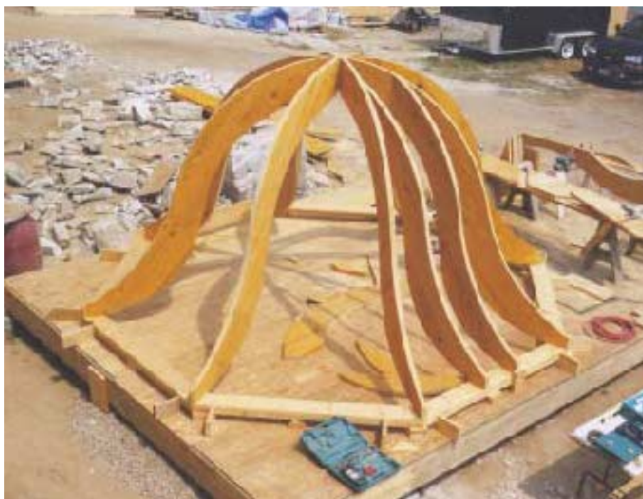
Figure 2. A temporary work platform served as a base for a double construction plate built to the exact dimensions of the existing wall plates. Stand-blocks maintain its position; 2-by blocks elevate the structure to aid the final lift.
