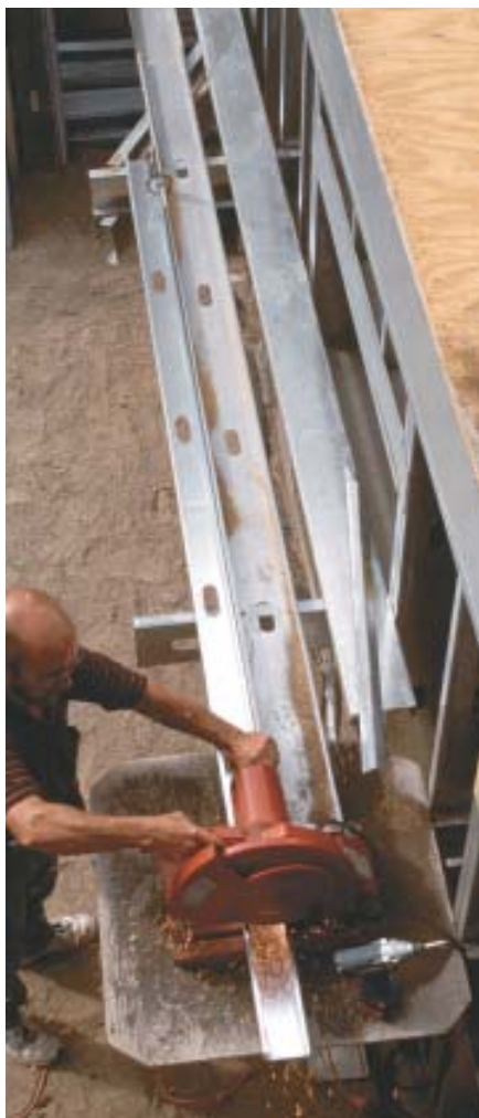
Figure 2. Most framers use chop saws with 14-inch abrasive blades to cut studs (right). It works, but the blades produce a lot of sparks and wear out quickly on heavier-gauge steel. It doesn't cost more to order precut studs, but if you need to cut on site, a dry-cut blade will do the job. The orange paint indicates that the joist is made from 14-gauge steel (below).
