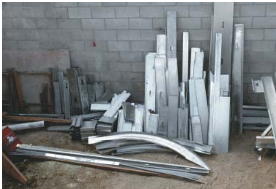
Figure 1. As you can see from the size of the scrap pile, there's not a lot of waste on a steel framing job. This is what's left after framing half of a 3,000-square-foot house.
