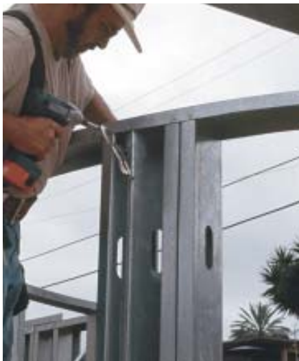
Figure 3. Wood frame carpenters are accustomed to framing walls flat and then standing them up. It's a little more work to do this with LGS because you have to flip the wall to fasten the other side (top). Traditionally, steel stud walls are assembled in the vertical position. The bottom track is fastened to the deck, the top track is propped up in the air, and the studs go in last (above and right). In this case, the supplier provided curved track for the curved walls.
