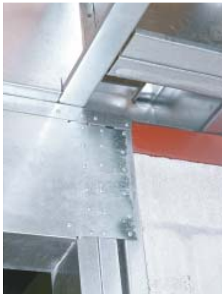
Figure 8. Jack studs aren't necessary in an LGS frame. In this case, the studs that make up the sides of the header are notched and the assembly is attached by screwing through the web.
