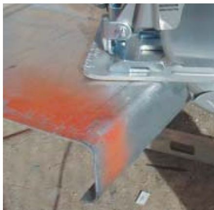
Figure 2. Most framers use chop saws with 14-inch abrasive blades to cut studs (right). It works, but the blades produce a lot of sparks and wear out quickly on heavier-gauge steel. It doesn't cost more to order precut studs, but if you need to cut on site, a dry-cut blade will do the job. The orange paint indicates that the joist is made from 14-gauge steel (below).
