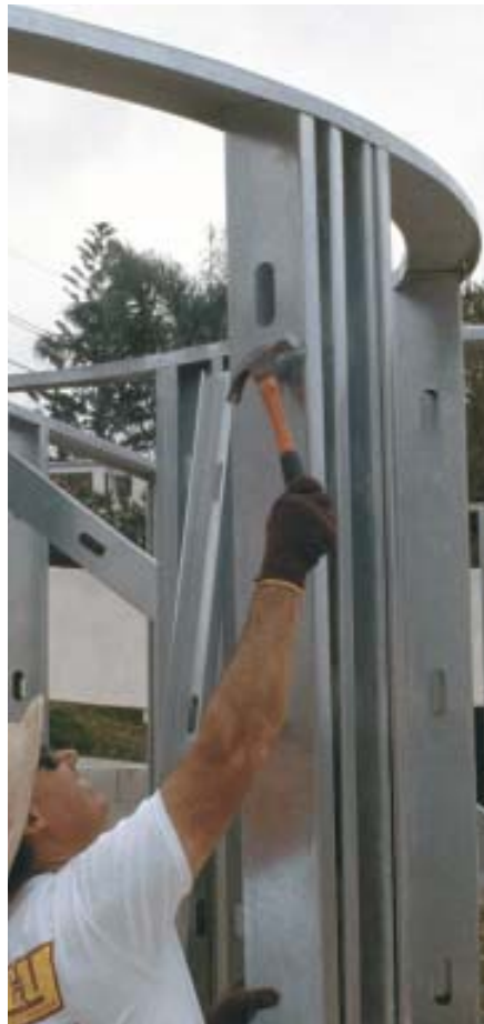
Figure 3. Wood frame carpenters are accustomed to framing walls flat and then standing them up. It's a little more work to do this with LGS because you have to flip the wall to fasten the other side (top). Traditionally, steel stud walls are assembled in the vertical position. The bottom track is fastened to the deck, the top track is propped up in the air, and the studs go in last (above and right). In this case, the supplier provided curved track for the curved walls.
