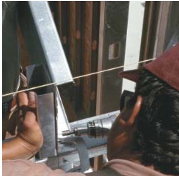
Figure 6. Web stiffeners are required at the bearing points of joists, rafters, beams, and headers. In this photo, the carpenter is using a short section of stud to stiffen the end of a rafter.
