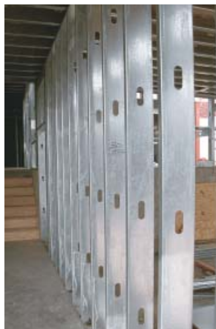
Figure 4. Studs, joists, and rafters are punched 2 inches on-center to accommodate pipes and wire. You should install them so the holes line up.
