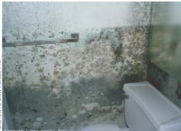
Figure 5. The bathroom is a naturally humid environment and is also prone to plumbing leaks that create continual wet conditions. Drywall, whether moisture resistant or not, supports thriving mold colonies in moist conditions. Use backerboard and tile instead, or a synthetic material like solid surfacing.
