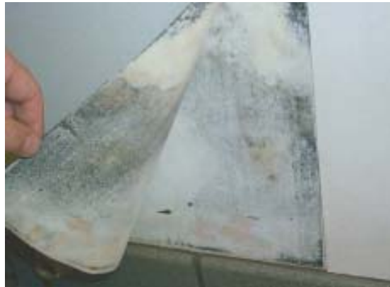
Figure 4. In hot, humid climates, vinyl wallpaper forms a vapor barrier on the cool, air-conditioned side of the wall, causing exterior moisture to accumulate under the wallpaper and support the growth of mold. Walls should be vapor-permeable on the side facing dry air, and vapor barriers should be placed on the side facing moist, warm air.
