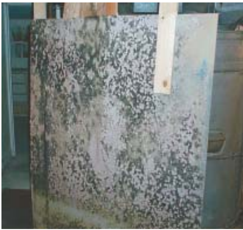
Figure 3. Damp basements are a friendly environment for mold. Extensive mold growth is visible on a drywall panel in a humid basement (left). The sawn lumber, which is less moisture absorbent and has less available nutrition for mold, has not been colonized. At right, high relative humidity has allowed mold to grow on engineered I-joist floor framing in a basement.
