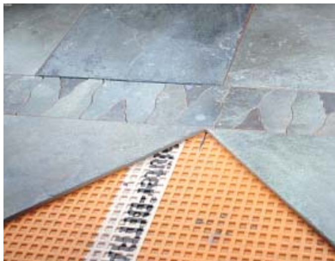
Figure 3. After covering the subfloor with a plastic uncoupling membrane, the author squares up the layout for an ornamental rug pattern (left). Full-sized tiles are dry-fitted in both directions from a line centered on the door mullion, followed by a 6-inch decorative tile band (lower left). A diagonal half-tile border sets up the diagonal field tiles in the pattern area (below).
