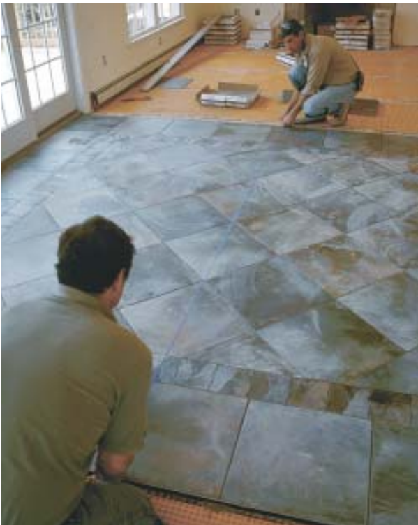
Figure 9. A line snapped across the points of the completed rug pattern permits accurate layout of the field areas to either side (left). Full half-diagonals initiate the general area installation (above).
