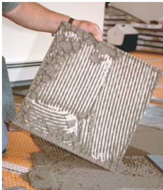
Figure 7. To prevent cracking, at least 95% of each tile should be contacting the thinset. The only way to check this is to pry up an occasional tile and look — but be careful not to crack the tile or dislodge the isolation membrane in the process.
