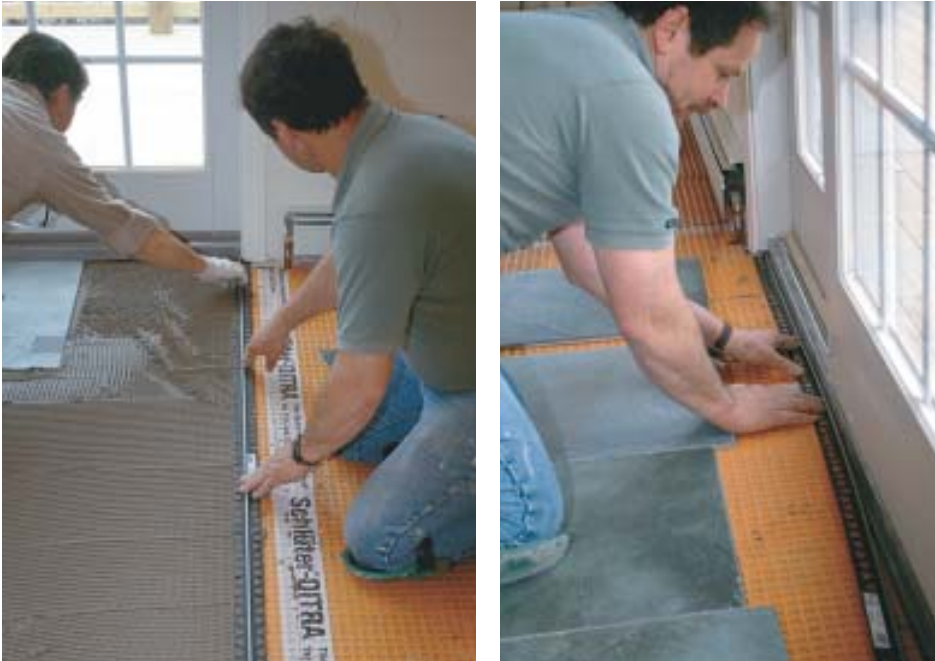
Figure 8. Large, uninterrupted expanses of tile should be divided into smaller sections with expansion joints to avoid stress cracks. The author uses a proprietary plastic strip that's available in a variety of colors for a good match with the grout (above left). Another strip, placed in front of the metal door sill, protects the adjoining grout and tile from damage caused by thermal expansion (above right).
