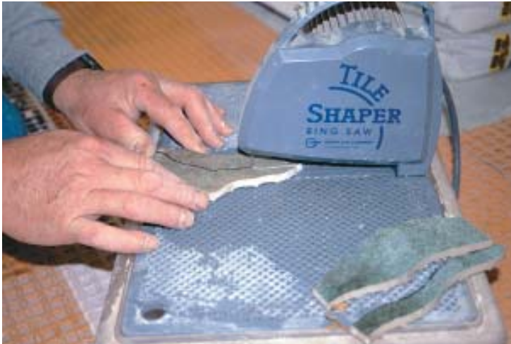
Figure 4. By expanding the border dimension of the rug pattern, the author created a space in the decorative tile layout too large for a single tile to fill yet too small for a full tile. Laying the cut-down tile at the border's corner effectively disguises the adjustment. A diamond-coated blade in a ring saw permits fast and accurate irregular cuts.
