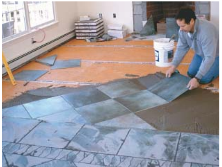
Figure 9. A line snapped across the points of the completed rug pattern permits accurate layout of the field areas to either side (left). Full half-diagonals initiate the general area installation (above).
