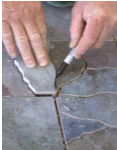
Figure 4. By expanding the border dimension of the rug pattern, the author created a space in the decorative tile layout too large for a single tile to fill yet too small for a full tile. Laying the cut-down tile at the border's corner effectively disguises the adjustment. A diamond-coated blade in a ring saw permits fast and accurate irregular cuts.
