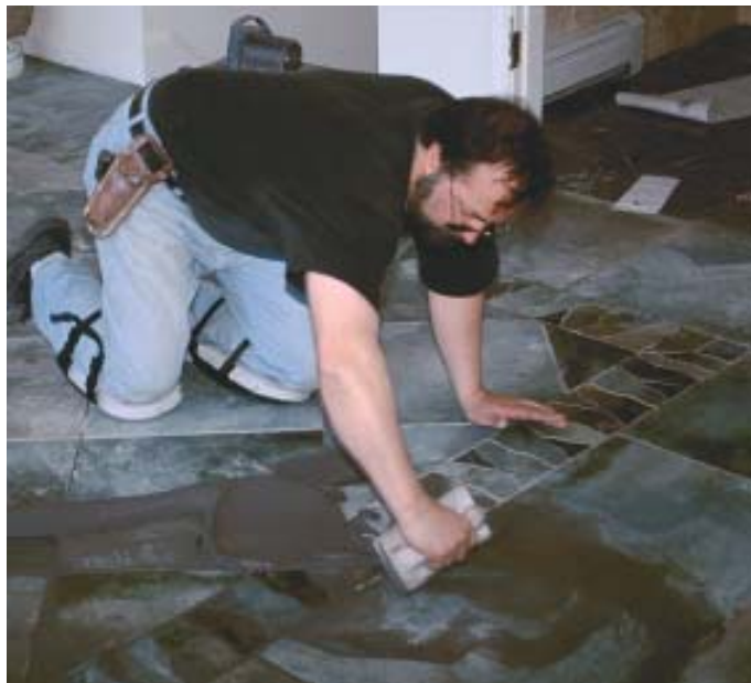
Figure 10. To prevent dried grout from sticking to the tile, spread only as much grout as can easily be cleaned within an hour (above). Clean water and regular rinsing with a sponge make for efficient cleanup. As the grout haze dries on the tile surface, the author and crew polish it away with soft rags and paper towels (right).
