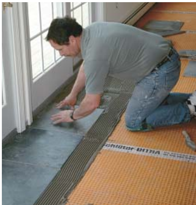
Figure 6. Combing the thinset adhesive in one direction with a notched trowel distributes the adhesive evenly and allows the tile to lie flat. Limiting thinset application to no more than 20 square feet at a time prevents the cement from drying prematurely.
