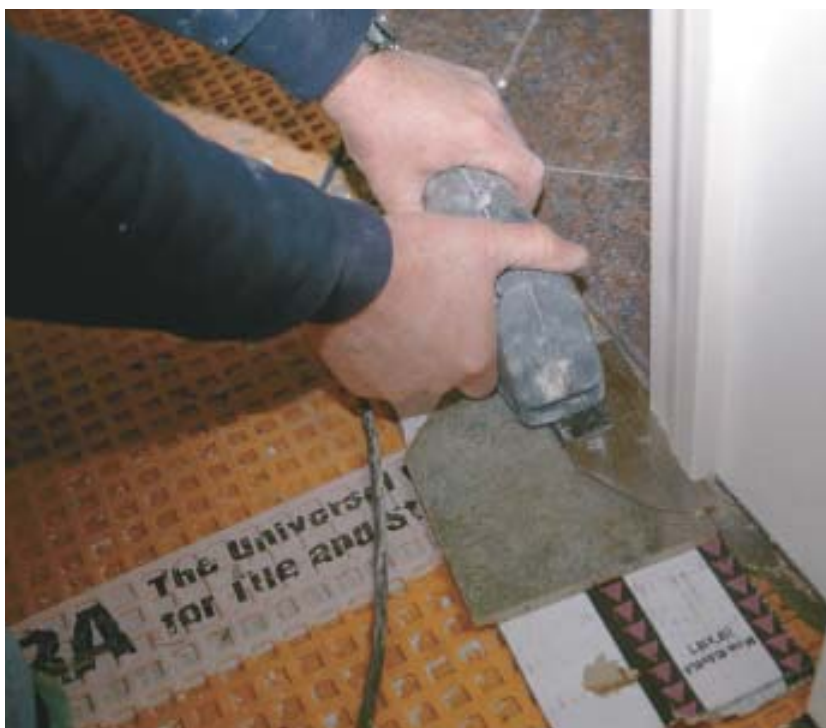
Figure 2. Rather than cutting tile around door casings, the author cuts a clear-space gap beneath with an undercut saw guided by a simple tile-and-cardboard gauge.
