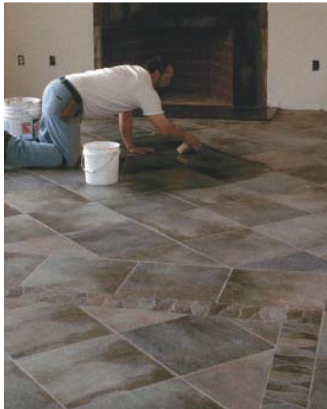
Figure 10. To prevent dried grout from sticking to the tile, spread only as much grout as can easily be cleaned within an hour (above). Clean water and regular rinsing with a sponge make for efficient cleanup. As the grout haze dries on the tile surface, the author and crew polish it away with soft rags and paper towels (right).
