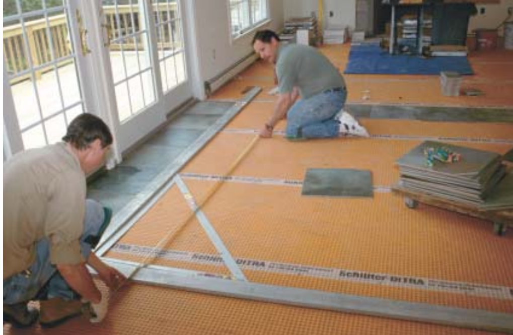
Figure 3. After covering the subfloor with a plastic uncoupling membrane, the author squares up the layout for an ornamental rug pattern (left). Full-sized tiles are dry-fitted in both directions from a line centered on the door mullion, followed by a 6-inch decorative tile band (lower left). A diagonal half-tile border sets up the diagonal field tiles in the pattern area (below).
