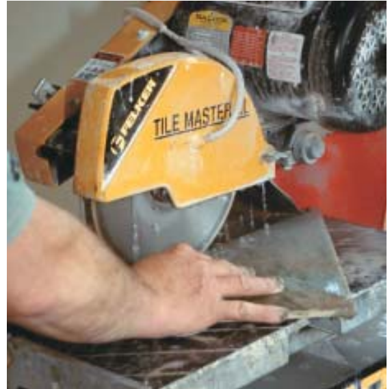
Figure 5. After drawing an accurate diagonal line on the tile, the author makes freehand cuts on a diamond-blade-equipped wet saw.
