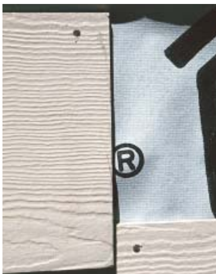
Figure 3. Blind-nailing is common with fiber-cement siding; the standard lap is 1\frac{1}{4} inches.
