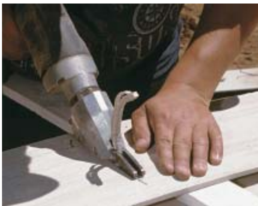
Figure 2. Electric shears, like this Snapper model, will cut fiber cement without producing dust. The downside is that they're slower than a circular saw and can cut only one piece at a time.
