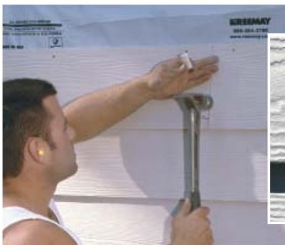
Figure 5. Wherever a butt joint doesn't lie flush because of irregular framing, the head of a single nail will close the gap and pull the pieces snug. This is less obtrusive than putting a nail in the corner of each piece.
