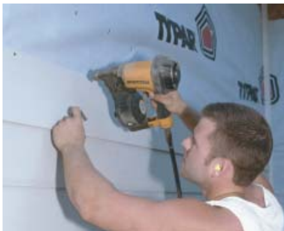
Figure 4. The author typically uses a roofing nailer because it fits easily under the eaves and in tight spots. Also, the large nail heads are hard to overdrive and hold siding flatter than nails with smaller heads.
