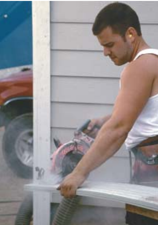
Figure 1. The author's crew gang-cuts as many as seven pieces at a time using a wormdrive saw (above). In contrast with a regular carbide blade, which would be dull after a single day of cutting, this dedicated fiber-cement blade from James Hardie has cut the siding for five 2,500-square-foot houses (right).
