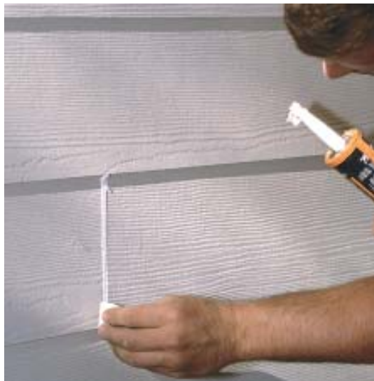
Figure 8. The author's crew always caulk as they go, so they won't have to clean the siding if it gets splattered with mud. Here, a carpenter uses a foam shipping block from a window to smooth the caulking at a butt.
