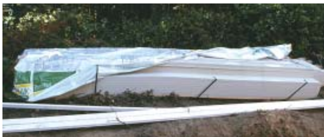
Figure 6. Have fiber-cement siding delivered to a spot where it's out of the way and won't have to be moved. This load weighed more than 4,000 pounds.
