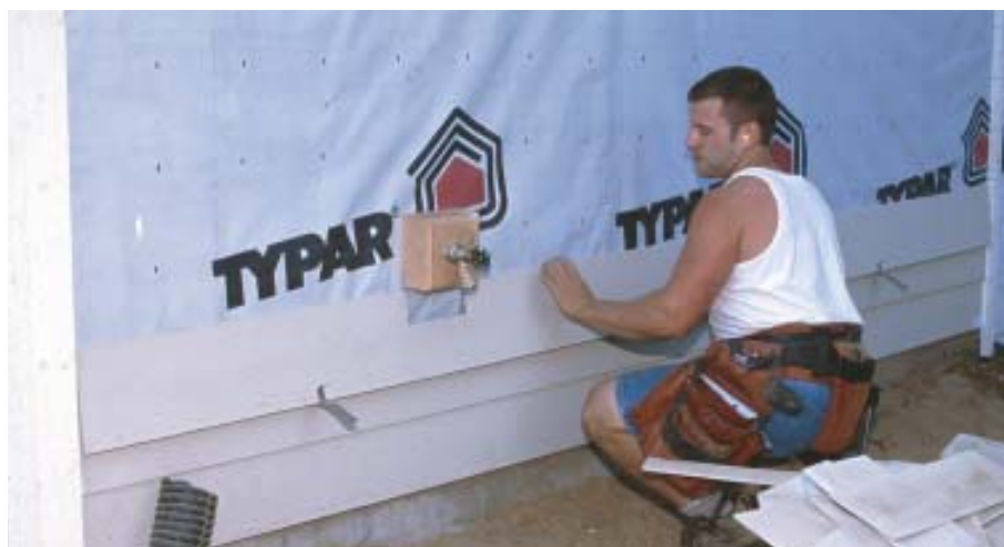
Figure 7. Because of its weight, fiber-cement siding is trickier to install when working alone than wood clapboards. Site-made or manufactured jigs, like the panel gauges shown here, are helpful. The gauges catch the upper edge of the previous course and hold the next piece in place while the carpenter nails it off.
