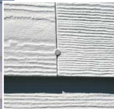
Figure 5. Wherever a butt joint doesn't lie flush because of irregular framing, the head of a single nail will close the gap and pull the pieces snug. This is less obtrusive than putting a nail in the corner of each piece.
