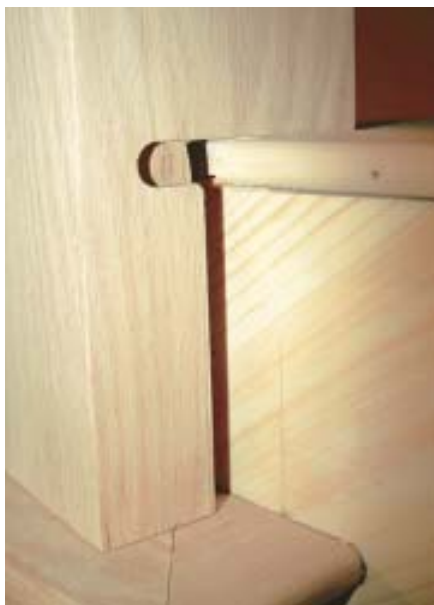
Figure 3. Newels at a landing are notched and fastened with hardened lag bolts (left). The recessed holes will later be plugged and sanded smooth. Where the newel is let into the stair nosing, the author provides a neat joint between post and tread by cutting an undersized notch and routing a matching profile in the face of the newel (right).
