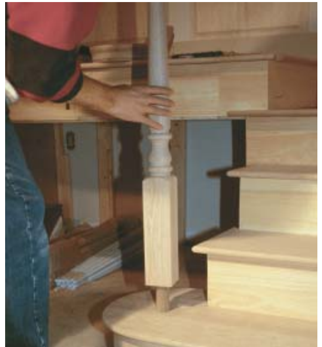
Figure 2. Adjustable starting newels are end-bored for an anchor dowel, which permits trimming them to length as needed (above left). Once the position of the starting newel has been determined with a paper template (left), the starting step is drilled through to the subfloor and the newel is dropped into place (above).
