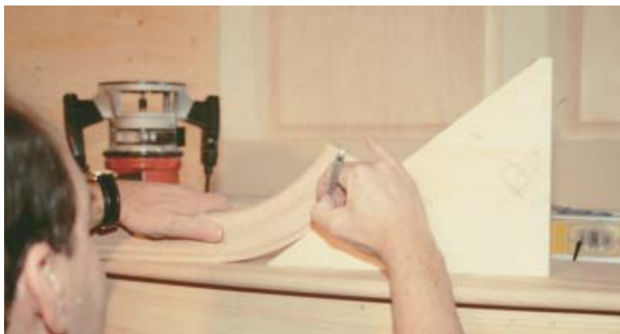
Figure 4. The correct cut location on a curved easing is established by positioning the pitch block beneath the curve and marking the tangent point (above). Rotating the block 90 degrees from its original position defines the cut line across the face of the easing (right).
