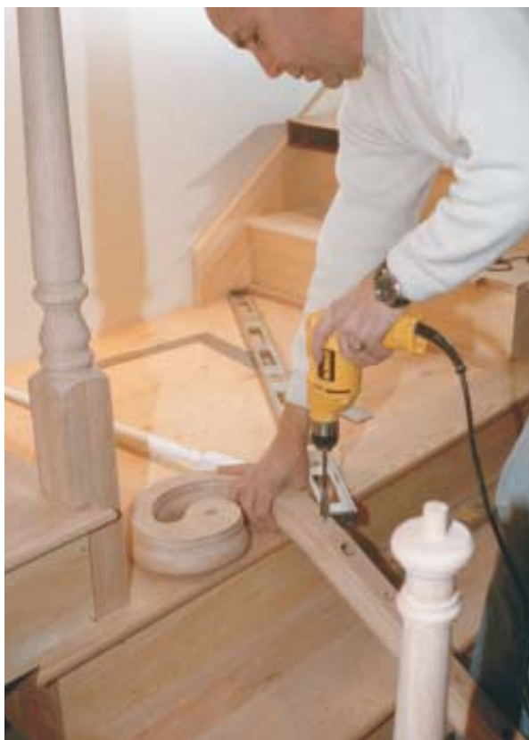
Figure 10. Drilling accurate holes for pin-top balusters is most easily done by turning the railing upside down on the stair. In that position, plumb holes will lie at the correct angle to the railing.
