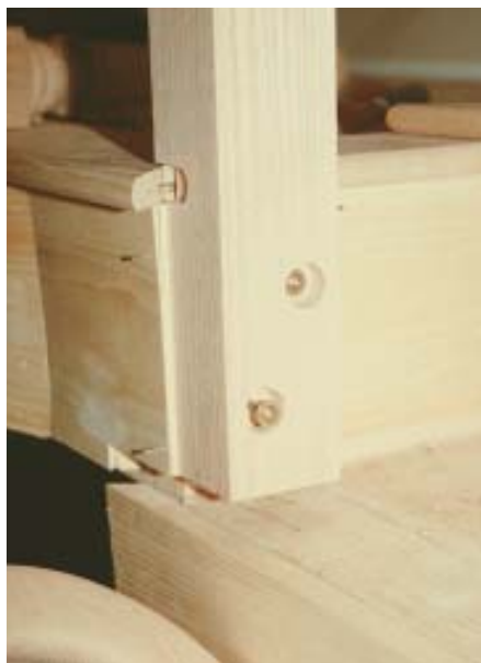
Figure 3. Newels at a landing are notched and fastened with hardened lag bolts (left). The recessed holes will later be plugged and sanded smooth. Where the newel is let into the stair nosing, the author provides a neat joint between post and tread by cutting an undersized notch and routing a matching profile in the face of the newel (right).
