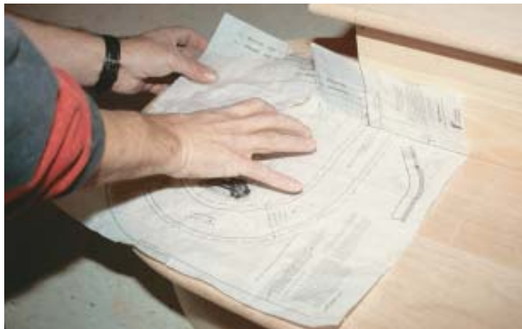
Figure 2. Adjustable starting newels are end-bored for an anchor dowel, which permits trimming them to length as needed (above left). Once the position of the starting newel has been determined with a paper template (left), the starting step is drilled through to the subfloor and the newel is dropped into place (above).
