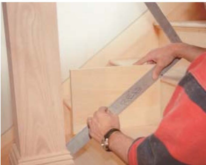
Figure 1. A pitch block is a simple gauge that's useful for determining post and rail height adjustments on offset newels. It's easily made by marking the diagonal between tread and riser on a square-cut lumber scrap (left), then cutting it to the line with a radial arm saw (right).
