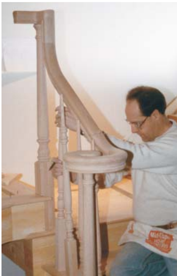
Figure 9. With the assembled railing dry-fitted to the newels, balusters are inserted and plumbed to establish the positions of the holes in the underside of the rail.
