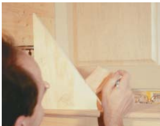
Figure 4. The correct cut location on a curved easing is established by positioning the pitch block beneath the curve and marking the tangent point (above). Rotating the block 90 degrees from its original position defines the cut line across the face of the easing (right).
