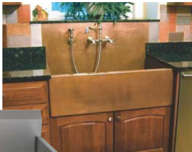
Figure 1. A high integral backsplash conceals wall-mount faucet supply lines and simplifies waterproofing the sink area.
