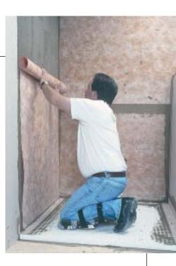
**Cementitious Backer Unit.** If cement board's your thing, you've got plenty of company. When installed over a waterproof membrane, cementitious backer unit (CBU) provides an unbeatable tile base in high-moisture applications. *PermaBase* is composed of Portland cement, lightweight aggregates including
