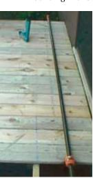
use two 10-footlong, <sup>3</sup>/4-inch black iron pipe clamps to squeeze all of the deck boards tight together. We place the clamps onefourth of the board length from the ends, checking the finished end for alignment and measuring at the clamps to be sure the courses are staying parallel. The ends of most deck boards are narrower than the middle from drying out, so clamping at the ends would create a bulge in the middle.
