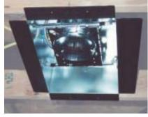
box hasn't compromised the fire rating. A better solution is to use the *e.z. barrier firebox*. The code-approved sheet-metal pan maintains the fire rating and eliminates the slow process of building and installing site-built barriers. This firebox works with 16- and 24-inch on-center spacing and costs \$42.
