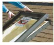
the opening from the exterior, making it unnecessary to go inside and check the reveal — a nice feature if you work by yourself. The snap-in sash also eliminates cladding removal and reinstallation process and the risk of lost fasteners or cladding parts. Available in 12 sizes, with widths from 16 to 44 inches and lengths from 27 to 72 inches, all
