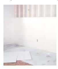
that won't support the growth of mold, reducing the chance of a serious problem. *DensArmor Plus*, with fiberglass on both sides, offers the best mold protection front and back, and reinforcing glass fibers in the gypsum core increase strength as well. Replacing stan-
