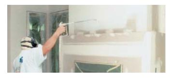
introduced spray-on product approaches the same level of finish in a shorter time. *Tuff-Hide*, a high-build spray-on primer, provides a high-quality base for paint finishes while eliminating joint telegraphing. When applied to the manufacturer's recommended application thickness of 15 to 20 mils, a gallon will cover approximately 125 square feet. The primer dries to the touch in 60 to 90 minutes. At the recommended thickness, Tuff-Hide costs about  $6\mathfrak{e}$  per square foot.
