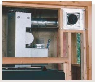
Installing a Replenum requires a 37-inch-tall, 24<sup>1</sup>/2-inch-wide, and 15-inch-deep cavity above the fireplace. The unit can be rotated on the flue collar to aid in positioning as long as a 2-inch air space from combustibles is maintained.
