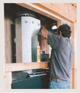
Keeping duct runs as straight as possible makes the recovery ventilator more efficient. The easiest way to accomplish this is straight through the back of the chase and straight through the interior wall, but the owner of this home wanted the exterior grill in a less obvious location, which required additional elbows.
