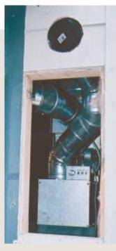
A 13x21-inch access panel is required for installation and servicing. The intake grill supplying the heat exchanger is located above the access panel, where it's less obtrusive. It's important to consider other exhaust vents, flues, and plumbing vents when locating the supply grill; otherwise, contaminated air could be drawn into the living space. The required clearances are included in the Replenum's wellwritten instructions.
