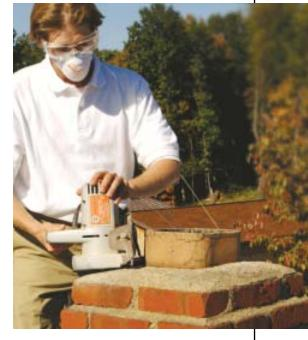
Water trapped between the chimney liner and the chimney pot can freeze, cracking the clay pot or the liner. Removing any flue tile that extends above the top of the chimney with a circular saw or grinder equipped with an abrasive or diamond blade prevents damage.
