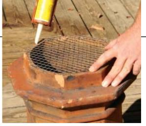
Before the pot is carried up to the roof, 1/2-inch wire mesh is cut to size and secured to the top of the chimney pot with silicone. The mesh acts as a spark arrester and keeps out animals and debris.
