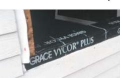
splitting the release paper into two parts much easier. With the paper split, you can adhere the membrane to the window opening and leave on the remaining release paper until it's time to install the housewrap or felt. The two-piece paper also aids in positioning the sticky membrane.
