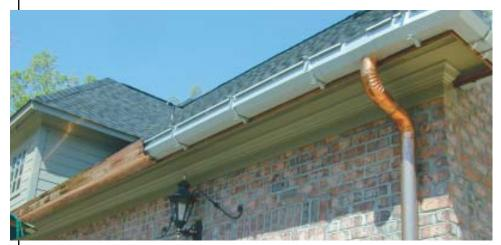
Once the cornice piece is installed, the gutter blends in with the trim. Sturdy, tightly spaced brackets and extra downspouts ensure that it can handle heavy rains without sagging or overflowing.
