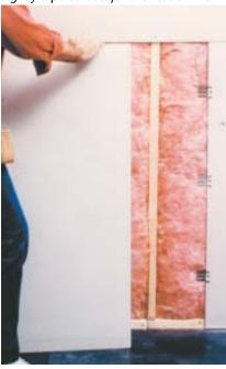
ing. Once the board is secured to the clips with screws, the front tab is broken off. Instabacks also make hanging ceilings easier by supporting one end of the board while you hold and fasten the other — great for solo work. They cost around 20¢ apiece in packages of 200.
