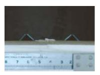
**Cover Your Butt.** No matter how skilled the finishing and feathering, even an untrained eye can pick up the hump of a butt seam in the right light, and today's big homes have more of them. Using the *Butthanger* is among the easier ways to deal with the problem. A U-shaped channel draws in the
