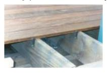
from Bangkerai, a Southeast Asian hardwood similar to Ipe. Two saw kerfs that run the length of the board receive a special T-shaped
