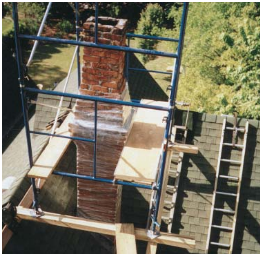
Figure 3. Solid, well-thought-out scaffolding provides a sense of security as well as a safe place to work. The chimney has been wrapped with plastic stretch wrap to help it resist the pressure of the fluid mortar that will be pumped around the inflatable formers.
