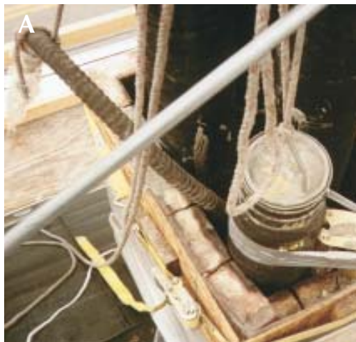
Figure 8. Once the inflatable flue formers have been inserted and properly positioned, liner mix will be carefully pumped into the chimney through the corrugated hose visible at right (A). Stainless-steel spring spacers wrapped around the flue formers prevent the formers from shifting as the flue mix is pumped between and around them (B and C). After the mix has set up overnight, the formers are deflated and withdrawn, leaving one or more smooth new flues (D).
