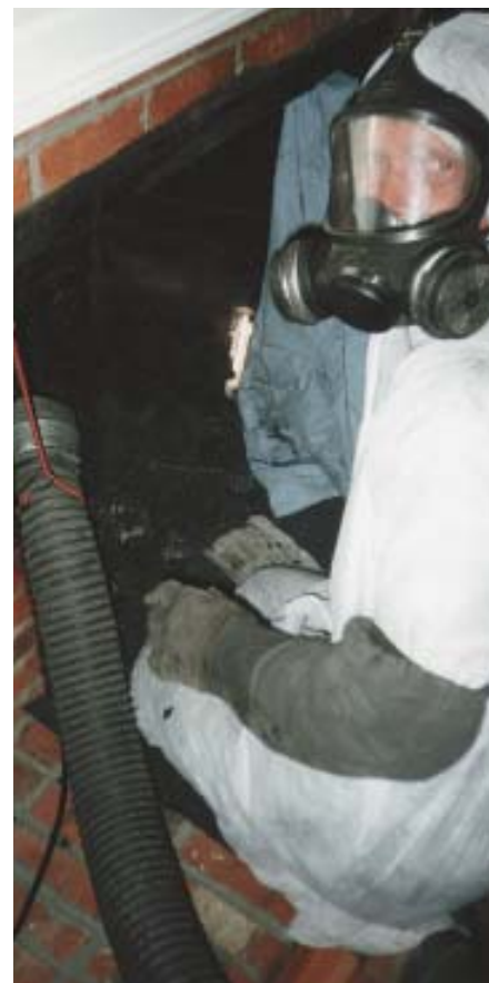
Figure 4. Tyvek coveralls and full-face respirators protect workers from potentially carcinogenic dust.
