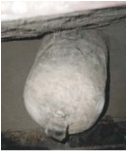
Figure 11. Once the temporary throat plate has been removed, the partially cured mass of material above the firebox is carefully carved away to expose the lower end of the flue former, creating a smooth, tapered smoke chamber.
