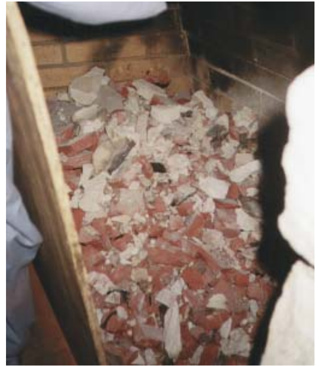
Figure 5. A plywood covering over the front of the fireplace contains broken masonry that falls from the chimney during demolition, and an efficient vacuum filters out dust before it can infiltrate the living space (above). The accumulated brick and mortar fragments are removed once the demo phase is complete (right).
