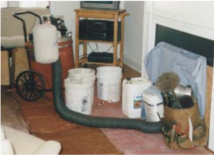
Figure 5. A plywood covering over the front of the fireplace contains broken masonry that falls from the chimney during demolition, and an efficient vacuum filters out dust before it can infiltrate the living space (above). The accumulated brick and mortar fragments are removed once the demo phase is complete (right).
