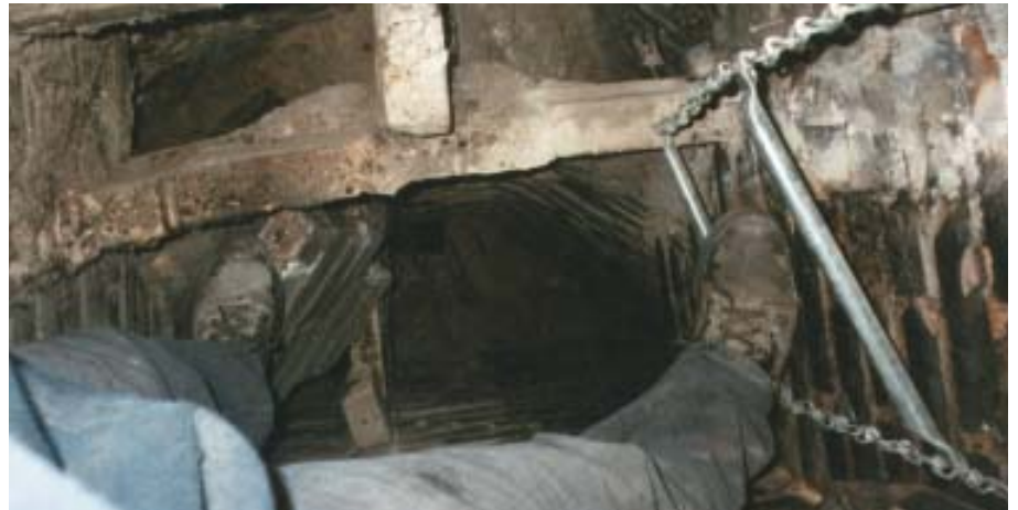
Figure 6. If the size of the chimney permits, a worker can climb into it from above to dislodge deteriorated wythes, providing the space needed for the new poured liner (above). A metal fire escape ladder fastened to the rooftop scaffolding provides safe and convenient access (left). Openings in the chimney wall, like the unused stovepipe thimble visible in the photo at left, must be bricked up before the liner is poured, or a disastrous blowout can result.
