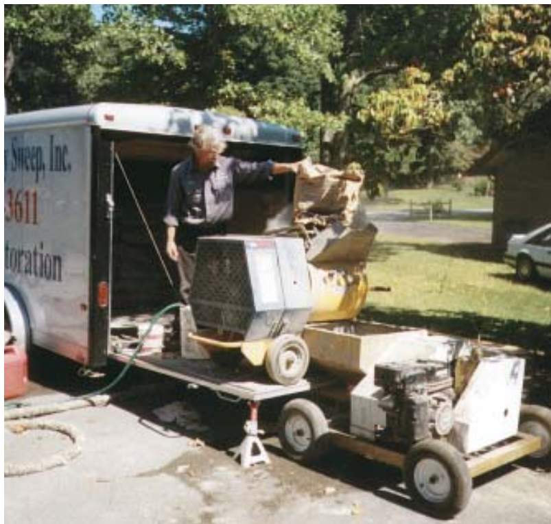
Figure 10. The proprietary flue mix is poured from a small mortar mixer into the hopper of the engine-powered pump that forces it to the rooftop. Workers on the roof and indoors remain in contact with the pump operator by walkie-talkie; if necessary, the pump can be reversed to suction the mix back into the hopper.
