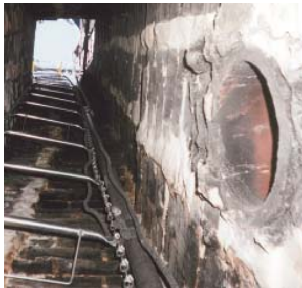
Figure 6. If the size of the chimney permits, a worker can climb into it from above to dislodge deteriorated wythes, providing the space needed for the new poured liner (above). A metal fire escape ladder fastened to the rooftop scaffolding provides safe and convenient access (left). Openings in the chimney wall, like the unused stovepipe thimble visible in the photo at left, must be bricked up before the liner is poured, or a disastrous blowout can result.
