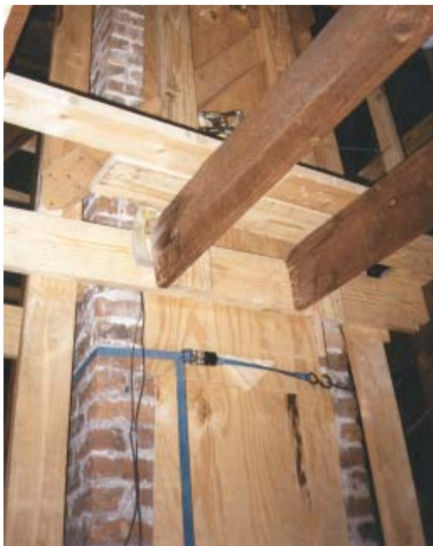
Figure 7. The freshly poured liner mix exerts considerable pressure on the surrounding brick, so tender old masonry is compressively reinforced with plywood and ratcheting cargo straps. Plywood and straps will be removed once the new poured liner has set up.
