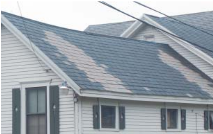
Figure 4. This repair with mismatched slates stands out like a sore thumb. If matching shingles were not available, the roofer could have repositioned existing slates while installing the new ones in a decorative pattern or band.
