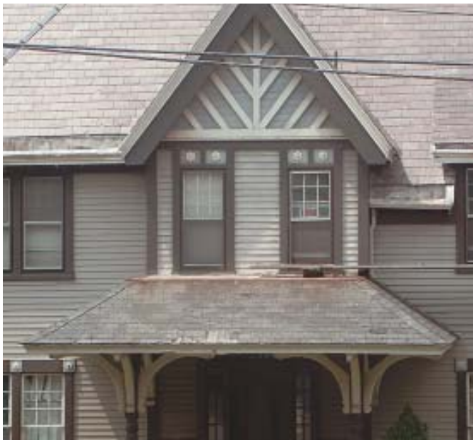
Figure 1. The main roof of this turn-of-the-century Victorian still has most of its original slates, while the asphalt shingles installed on the building's lower porch roof in mid-century are at the end of their service life.
