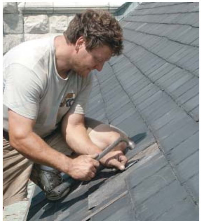
Figure 7. Removing a cracked slate is quick and simple with a slate ripper: The roofer slides the tool under the slate and hooks the slate out with a combined pulling and levering action (top left and right). A slate hook driven into the roof will hold the bottom of the replacement slate (bottom right). Sometimes the installer needs to punch and grind a pilot hole for the hook into the crack between the two slates in the course below (bottom left).
