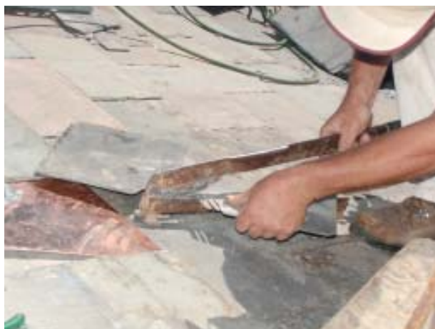
Figure 6. A slate cutter's lever arm is powerful enough to readily shear through slate but allows fine control for careful cutting. Here, slate roofing contractor John Kuhn uses the tool to nibble out a half circle for a vent pipe penetration.
