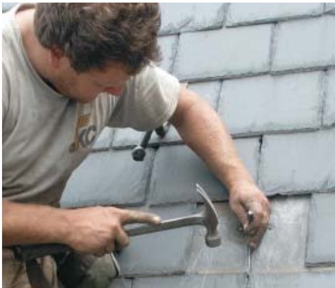
Figure 7. Removing a cracked slate is quick and simple with a slate ripper: The roofer slides the tool under the slate and hooks the slate out with a combined pulling and levering action (top left and right). A slate hook driven into the roof will hold the bottom of the replacement slate (bottom right). Sometimes the installer needs to punch and grind a pilot hole for the hook into the crack between the two slates in the course below (bottom left).
