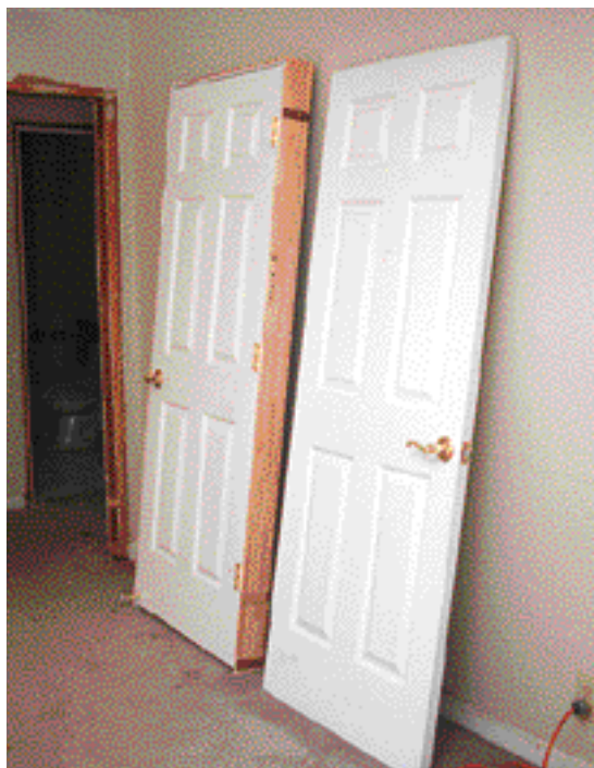
Figure 3. Interior doors are always in strong demand. They're easily freed by removing the casing and cutting the nails with a recip saw. Driving a nail through the jamb holds the door closed and leaves it ready for a new life in another house.
