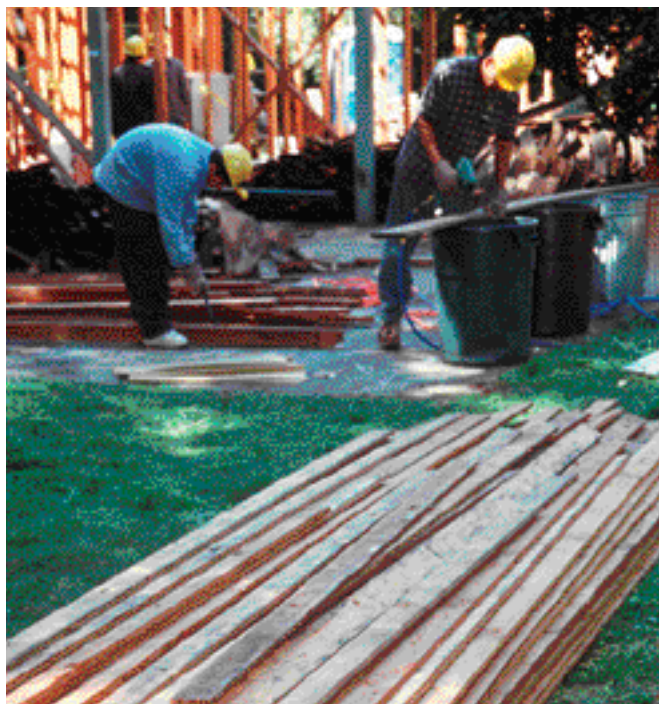
Figure 2. It's not economical to salvage short pieces of framing lumber or sheathing, but longer material readily finds buyers. This 1x4 skip sheathing was sold from the site, along with most of the 2-by framing stock.
