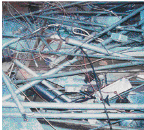
Figure 4. Although there's a lot of metal in an old house, little of it is salvageable. But if it's all collected in one place, at least you don't have to pay to get rid of it. The author collects metal in a separate dumpster that a metal recycling company hauls away for free.
