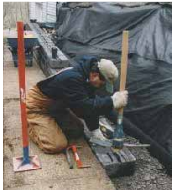
Figure 4. The author likes to firmly bed his base course of block into the granular base by beating the block with the top of the pick handle (right). He prefers to use the heavy Versa-Lok units shown here because in his experience they stand up to this treatment better. The depth of the first course of block ("toe embedment") varies depending on site characteristics (above). If the ground slopes downhill from the wall base, manufacturer specs call for a deeper embedment to hold the base in place.
