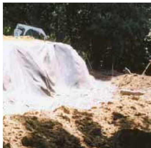
Figure 2. The author always checks site soils carefully to identify uncompacted fill or problem soils. The upper left photo shows fill on the site of an existing 40-year-old home. The material is a silty sand that drains well. The author excavated down to original virgin soil for his wall base and placed filter fabric over the bank to keep fines out of the drain system (above). The photo at left shows a nearly vertical cut bank of native clay soils where contractor Jason Sweeney excavated the hillside to make room for a pool. Drainage is particularly important behind this wall, because the clay becomes soft and heavy when wet.
