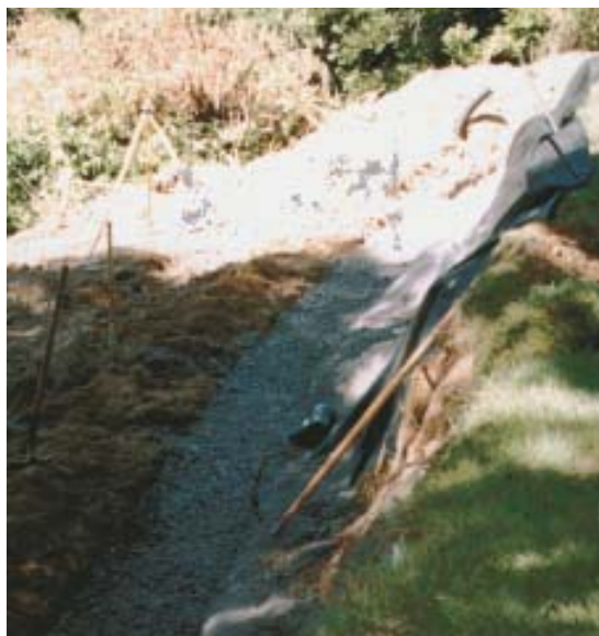
Figure 3. A base of "crusher run," ground stone and stone dust, is placed in the footing trench and tamped hard to support the base course of block. The taller the wall or the less firm the subgrade soils, the deeper and wider the base of crusher run should be.
