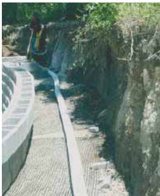
Figure 2. The author always checks site soils carefully to identify uncompacted fill or problem soils. The upper left photo shows fill on the site of an existing 40-year-old home. The material is a silty sand that drains well. The author excavated down to original virgin soil for his wall base and placed filter fabric over the bank to keep fines out of the drain system (above). The photo at left shows a nearly vertical cut bank of native clay soils where contractor Jason Sweeney excavated the hillside to make room for a pool. Drainage is particularly important behind this wall, because the clay becomes soft and heavy when wet.
