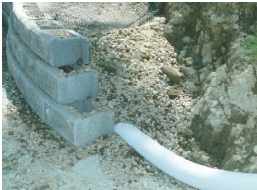
Figure 5. A drain tile in the granular backfill, sloped and run to daylight, is critical for retaining wall performance. It helps keep frost problems to a minimum and maintains soil behind the wall in a drained condition to reduce lateral pressure of soil against the wall.
