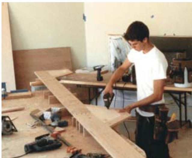
Figure 7. Some arches were wider than the length of available alder stock. These sections have pocket-screw joints at mid span.
