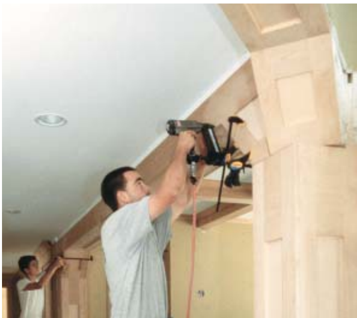
Figure 7. Some arches were wider than the length of available alder stock. These sections have pocket-screw joints at mid span.
