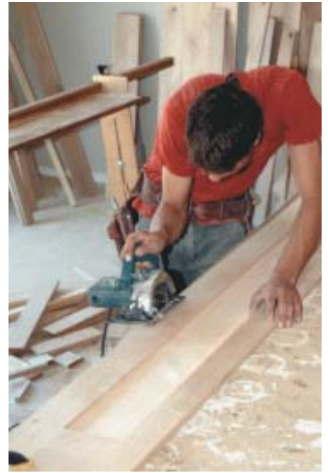
Figure 4. Pilaster columns are scribed to the wall (left), then trimmed to the line with a Makita panel saw (right), held to cut a slight back-bevel for a tight fit at the wall.
