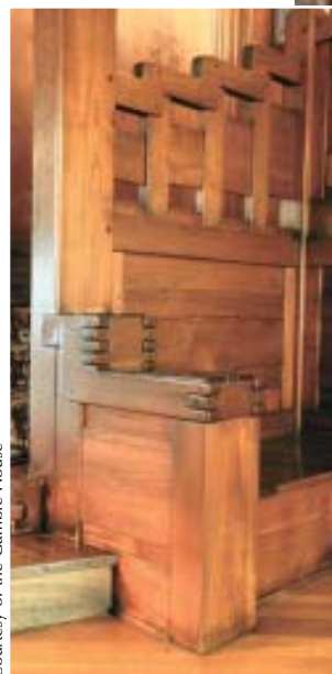
Figure 8. The column plinths were assembled from \frac{3}{4} -inch alder-veneer plywood. Baseboard followed flooring. The finished paneling is reminiscent of early 20th-century Craftsman-style woodwork (inset).
