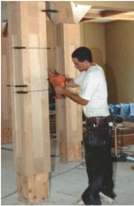
Figure 3. Clamps hold the glued panels in place while a carpenter secures the joints and the field with finish nails.
