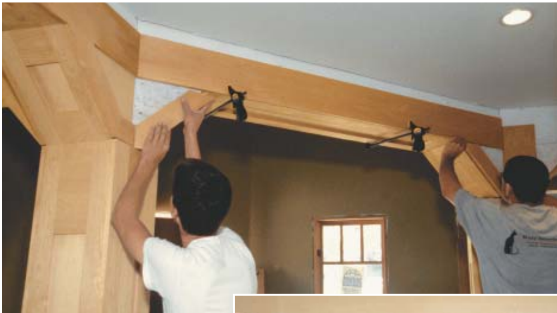
Figure 6. Some of the columns have miters in two directions, requiring careful dry-fitting (above). Even the 1/4-inch panels are mitered (right).
