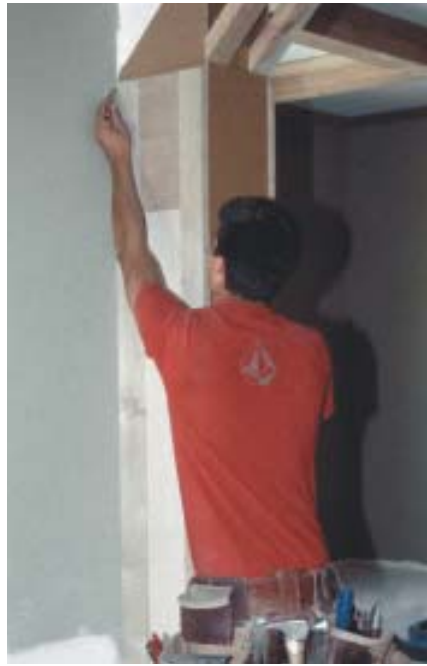
Figure 4. Pilaster columns are scribed to the wall (left), then trimmed to the line with a Makita panel saw (right), held to cut a slight back-bevel for a tight fit at the wall.
