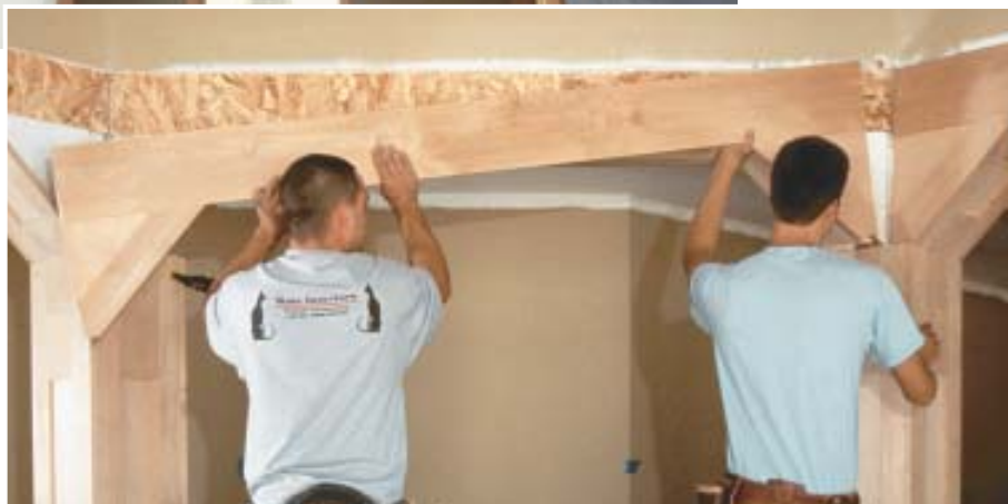
Figure 6. Some of the columns have miters in two directions, requiring careful dry-fitting (above). Even the 1/4-inch panels are mitered (right).
