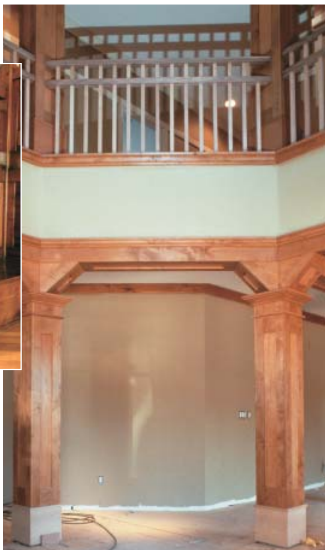
Figure 8. The column plinths were assembled from \frac{3}{4} -inch alder-veneer plywood. Baseboard followed flooring. The finished paneling is reminiscent of early 20th-century Craftsman-style woodwork (inset).
