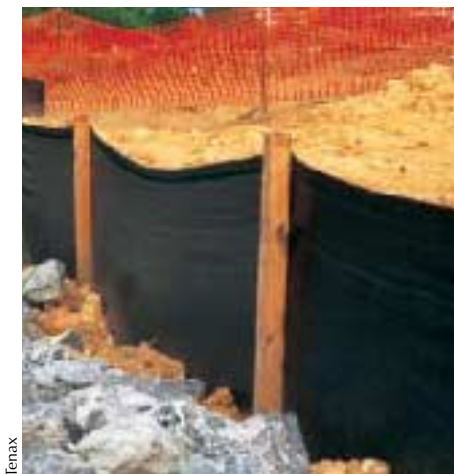
Figure 2. Geotextiles have become a commodity product, with many companies competing to provide choices across the whole range of strength, porosity, and other properties. Silt fences (left) and filter wraps for trench drains (right) are familiar uses to most builders.
