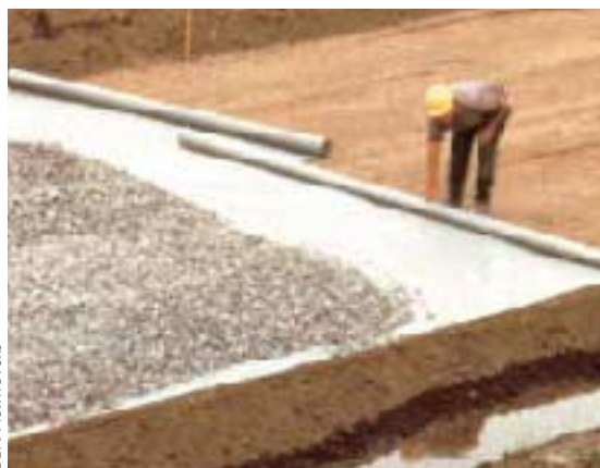
Figure 3. For roads ranging from temporary access roads to super-highways, tough woven fabrics isolate the gravel road base from soft soil subgrades, stabilizing the road structure and dramatically prolonging its life.
