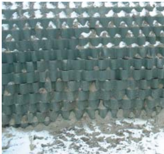
Figure 6. Cellular confinement systems, or geocells, lend great strength to roadbeds and embankments in heavy engineered applications. Gravel-filled Presto Geoweb geocell material provides a solid roadbed (top), while soil-filled Tenax Tenweb stabilizes a bank (above). Stacks of filled Terrafix Terraweb form a strong earth-retaining wall (left).
