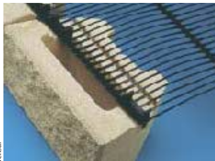
Figure 5. Tough, large-weave plastic geogrids are used primarily for structural soil reinforcement. One important use in residential work is to tie together the soil mass of a segmental block retaining wall structure. Although the grids typically interlock with the individual block (above), they function mainly to lock the soil into a stable mass, not to tie back the block. With internal soil pressures managed by the geogrid reinforcement, segmental block walls can readily reach 30 feet or more in height (right).
