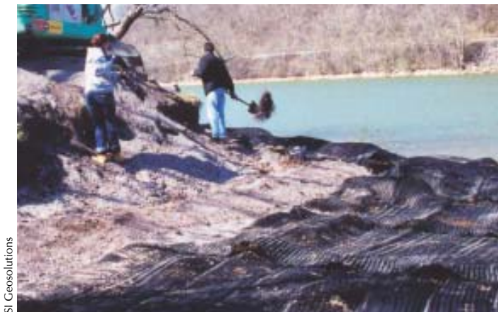
Figure 4. Tangled open-weave fabrics made from heavy plastic strands (right) provide a tough anchorage for plants to resist stormwater erosion and trap silt. Wrapping heavy fabrics around soil on an exposed river or lake bank can hold the bank in place and help plants stay anchored (below).
