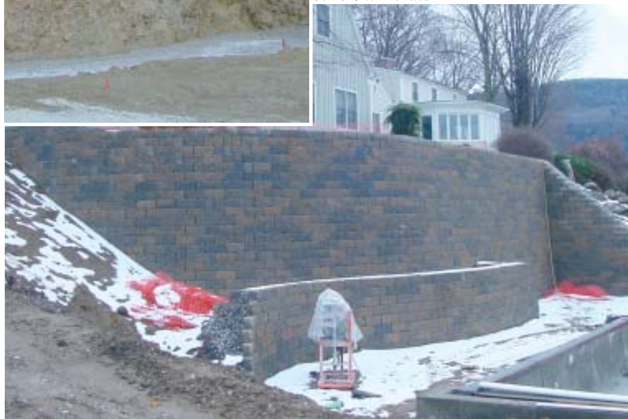
Figure 5. Tough, large-weave plastic geogrids are used primarily for structural soil reinforcement. One important use in residential work is to tie together the soil mass of a segmental block retaining wall structure. Although the grids typically interlock with the individual block (above), they function mainly to lock the soil into a stable mass, not to tie back the block. With internal soil pressures managed by the geogrid reinforcement, segmental block walls can readily reach 30 feet or more in height (right).
