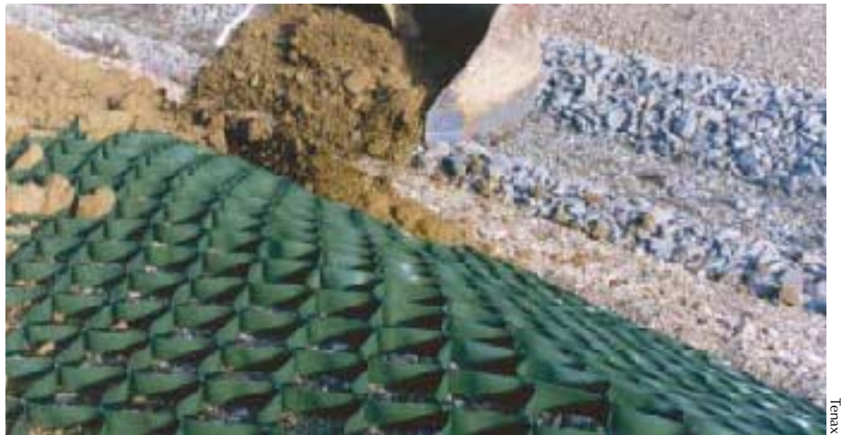
Figure 6. Cellular confinement systems, or geocells, lend great strength to roadbeds and embankments in heavy engineered applications. Gravel-filled Presto Geoweb geocell material provides a solid roadbed (top), while soil-filled Tenax Tenweb stabilizes a bank (above). Stacks of filled Terrafix Terraweb form a strong earth-retaining wall (left).
