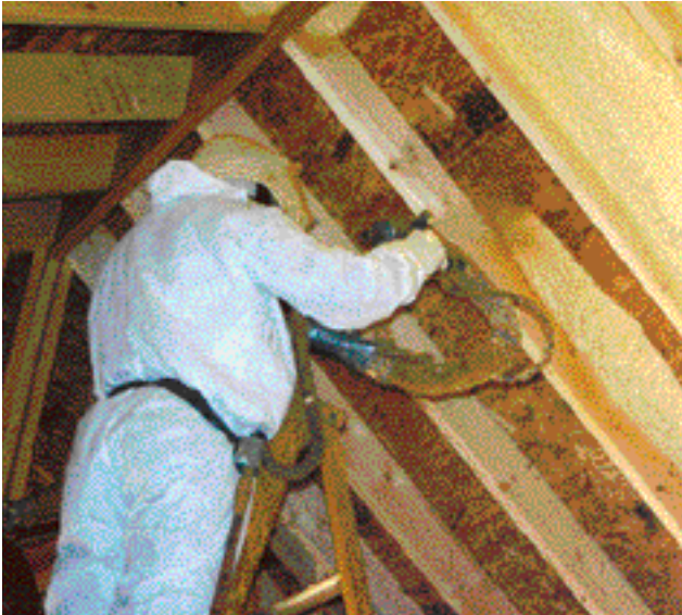
Figure 3. Spray-applied foam insulation allows you to build cathedral ceilings without venting or vapor barriers. It also allows you to build unvented attics.
