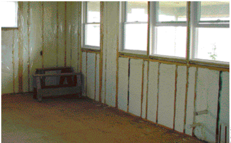
Figure 2. Open-cell foam is more permeable to vapor than closed-cell material. All foam is designed to be used without a vapor barrier, but some inspectors will make you use it, as in this kitchen that was insulated with 1/2-pound foam.
