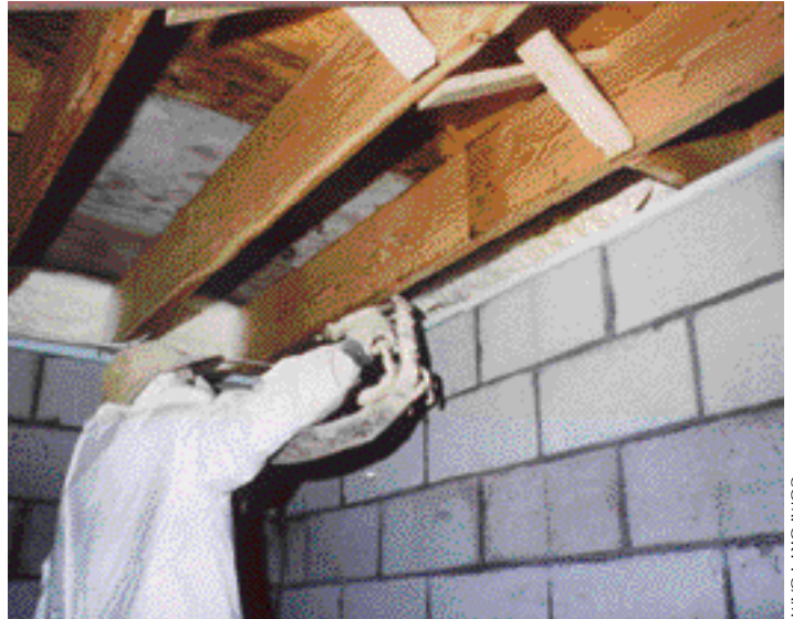
Figure 4. Rim joists are difficult to insulate and nearly impossible to fully seal with traditional insulation and vapor barriers. Foam allows you to do a much better job insulating areas that are often poorly done.
