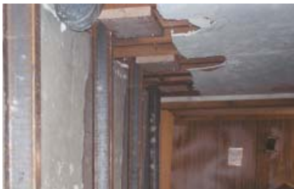
Figure 9. The completed I-beam installation (right) supplies reinforcing for the wall from footing to sill at 3 to 6 feet on-center. In the example below, the author then applied fiber-reinforced plastic panels to the basement walls. The basement is now ready for further finishing.
