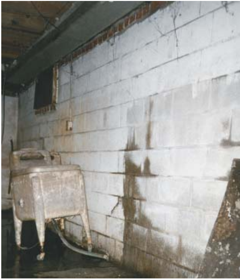
Figure 2. Block basement walls (above) tend to bulge in the center. Poured walls (right) are more likely to lean inward at the top due to failure of the sill connection. I-beams can stabilize both types of wall in place as long as the deflection is no greater than 3 inches. Block walls that are more than 3 inches out should probably be rebuilt. Poured walls that are more than 3 inches out can be pushed back to plumb and then stiffened with I-beams. For jobs requiring rebuilding or pushing back walls, exterior soils must be excavated, but for simple stabilization jobs, regrading may be sufficient.
