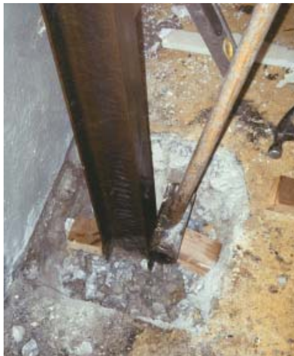
Figure 6. The author braces the base of each I-beam in place with small blocks of wood. The wood blocks will be encased in the concrete pier base when the hole is grouted.
