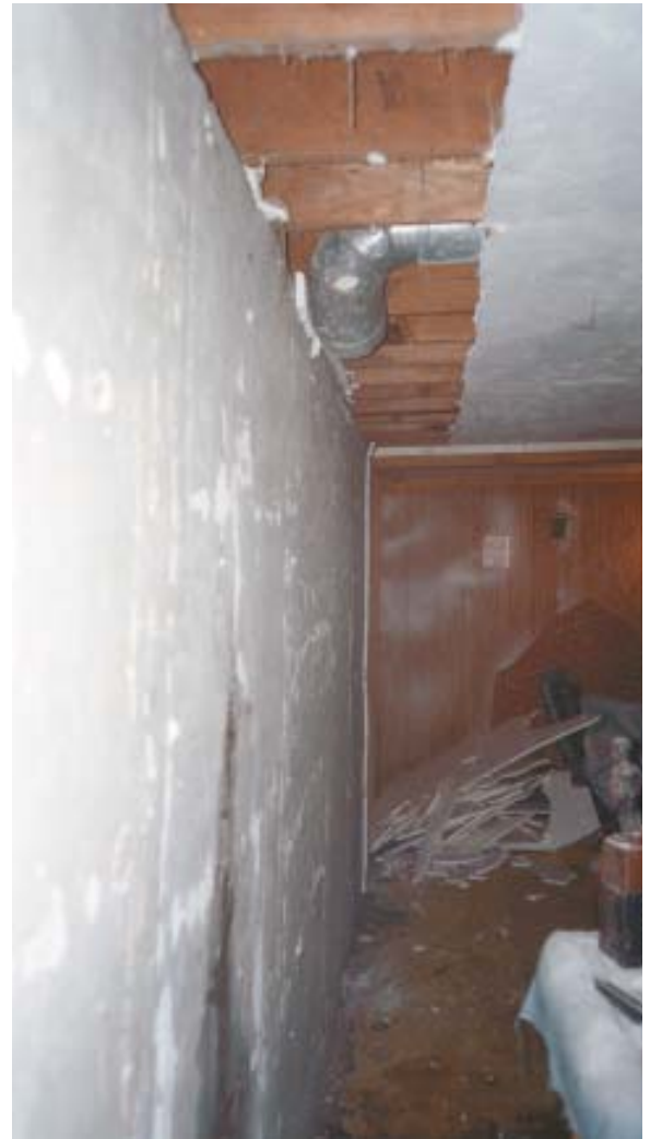
Figure 2. Block basement walls (above) tend to bulge in the center. Poured walls (right) are more likely to lean inward at the top due to failure of the sill connection. I-beams can stabilize both types of wall in place as long as the deflection is no greater than 3 inches. Block walls that are more than 3 inches out should probably be rebuilt. Poured walls that are more than 3 inches out can be pushed back to plumb and then stiffened with I-beams. For jobs requiring rebuilding or pushing back walls, exterior soils must be excavated, but for simple stabilization jobs, regrading may be sufficient.
