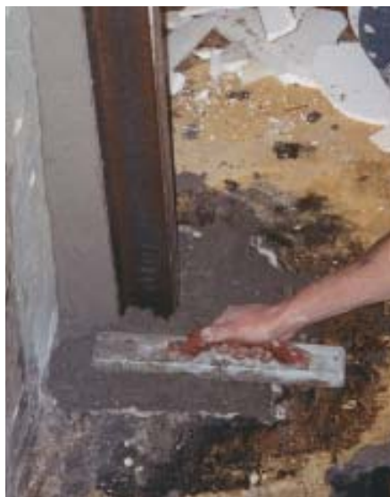
Figure 8. The hole is filled with stiff concrete to embed the I-beam firmly into the slab and subbase. The surface is troweled level with the existing slab.
