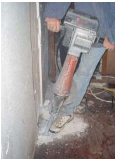
Figure 3. After cutting back the insulating foam, a worker jackhammers through the floor slab and footing edge. A steel I-beam will be placed in each hole and set in concrete. The author prefers jackhammering to concrete sawing, because it creates less dust and provides a rough edge for good bonding between the existing concrete and the freshly placed pier footing.
