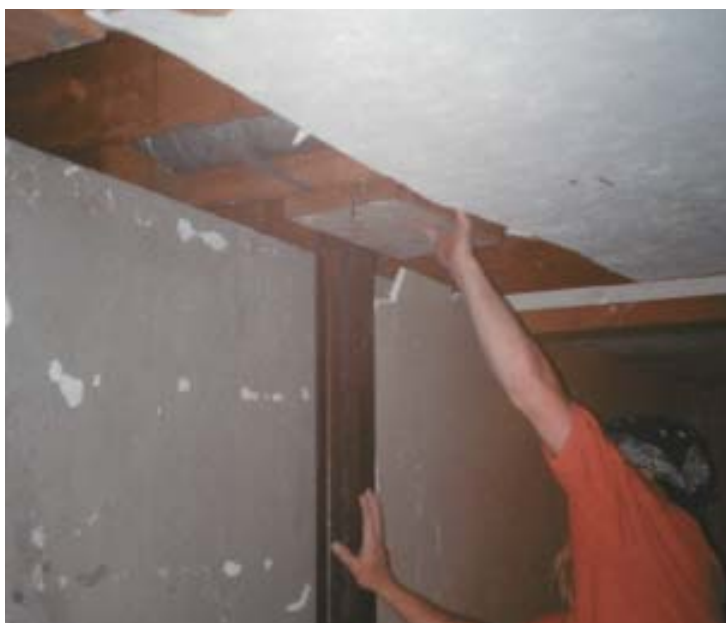
Figure 4. A worker braces the top of an I-beam tight against the top of the leaning wall (left). The 2x10 brace is fastened to the existing floor joists using 3/8-inch lag bolts sunk into predrilled holes (right). Three-inch by three-inch angle iron can be used instead of the 2x10 block. This step is easier with two people — one to hold the I-beam and block in place, and one to set the lag bolts.
