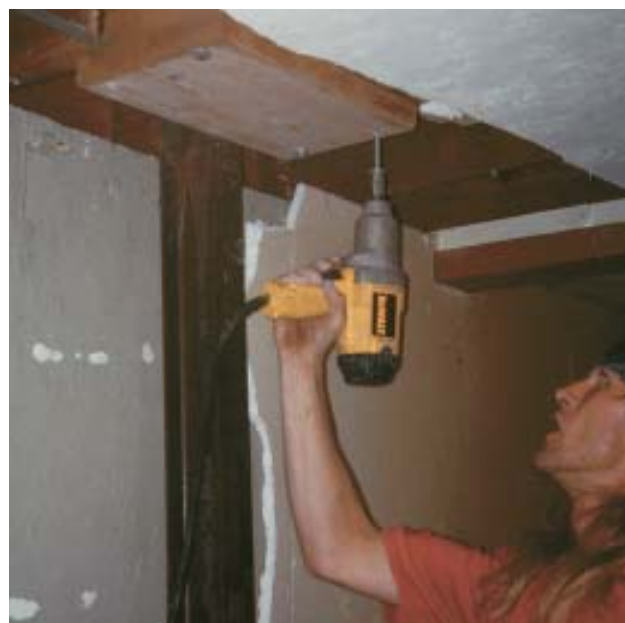
Figure 4. A worker braces the top of an I-beam tight against the top of the leaning wall (left). The 2x10 brace is fastened to the existing floor joists using 3/8-inch lag bolts sunk into predrilled holes (right). Three-inch by three-inch angle iron can be used instead of the 2x10 block. This step is easier with two people — one to hold the I-beam and block in place, and one to set the lag bolts.
