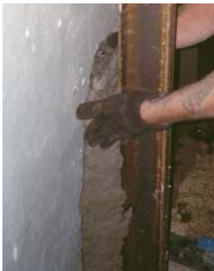
Figure 7. A worker grouts the entire space between the I-beam and the wall with stiff concrete to provide full support for the wall. Excess grout is smoothed away for a clean finish (see photo on page 75).
