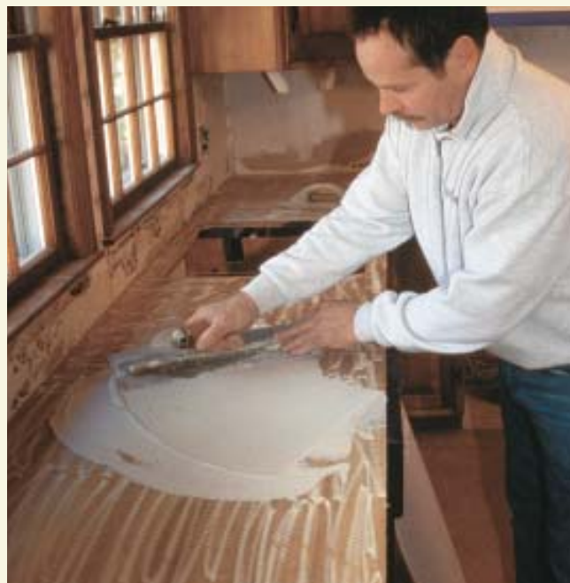
Figure 1. The existing laminate countertop is roughed up with an electric grinder to provide a good bonding surface (above). There's no need to leave grind marks on every square inch, but the entire surface should be liberally scratched up (above right). A uniform coating of latex-modified thinset cement is then spread and combed out with a V-notch trowel (right).
