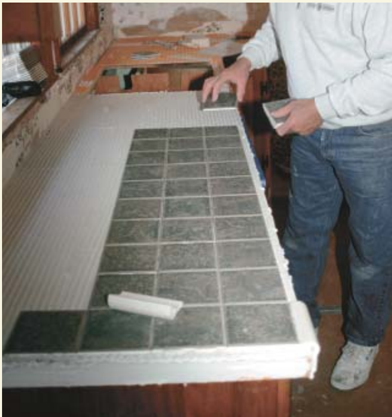
Figure 4. Full tiles are set from an outside corner of the layout toward the sink cutout. Installing a piece of nosing against one edge of the corner tile determines how much the remaining tiles should be held back from the edge to accommodate the remaining nosing (above). Nosing pieces are subject to hard knocks, so they're generously back-buttered to ensure that they're thoroughly embedded (right).
