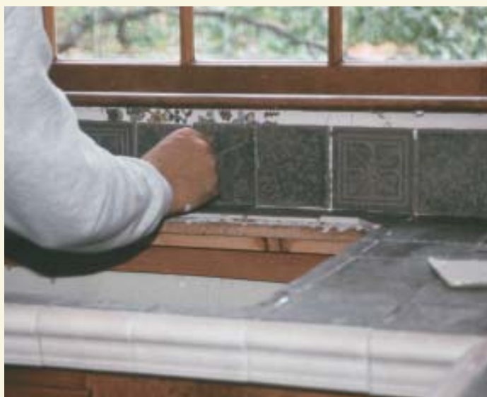
Figure 5. To prepare the wall-papered wall for a tile backsplash — which will be fastened directly to the wall-board — the author first coats the area with a water-based mastic (above left). Poorly bonded areas of wallpaper bubble away from the wall-board and are easily scraped off with a small trowel, leaving an acceptable tile base (above right). The backsplash tiles are then attached to the wall with more mastic (left).
