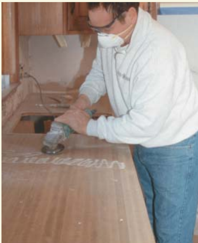
Figure 1. The existing laminate countertop is roughed up with an electric grinder to provide a good bonding surface (above). There's no need to leave grind marks on every square inch, but the entire surface should be liberally scratched up (above right). A uniform coating of latex-modified thinset cement is then spread and combed out with a V-notch trowel (right).
