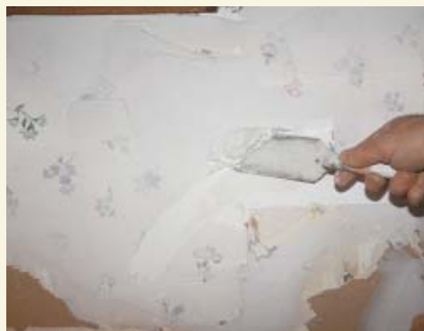
Figure 5. To prepare the wall-papered wall for a tile backsplash — which will be fastened directly to the wall-board — the author first coats the area with a water-based mastic (above left). Poorly bonded areas of wallpaper bubble away from the wall-board and are easily scraped off with a small trowel, leaving an acceptable tile base (above right). The backsplash tiles are then attached to the wall with more mastic (left).
