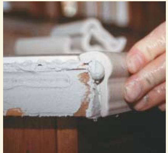
Figure 4. Full tiles are set from an outside corner of the layout toward the sink cutout. Installing a piece of nosing against one edge of the corner tile determines how much the remaining tiles should be held back from the edge to accommodate the remaining nosing (above). Nosing pieces are subject to hard knocks, so they're generously back-buttered to ensure that they're thoroughly embedded (right).
