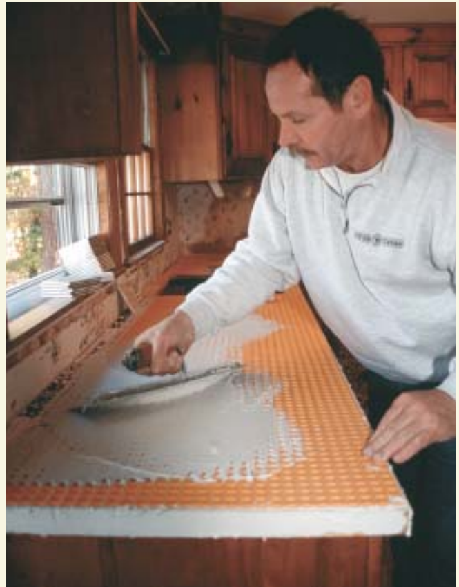
Figure 3. Once the tile layout has been fine-tuned (left), more thinset is troweled into the waffle-patterned surface and onto the exposed edges of the countertop, which were previously stripped of their laminate self-edging (below).
