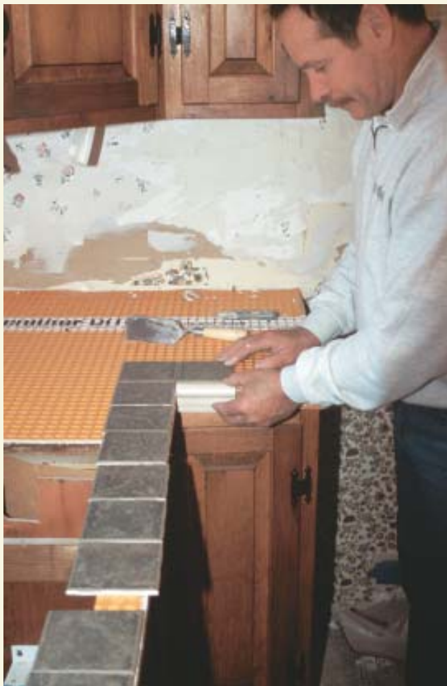
Figure 3. Once the tile layout has been fine-tuned (left), more thinset is troweled into the waffle-patterned surface and onto the exposed edges of the countertop, which were previously stripped of their laminate self-edging (below).
