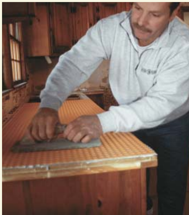
Figure 2. Precut sheets of textured polyethylene membrane go on over the cement (above left) and are bedded firmly in place with a wood float (above). An edge view of the proprietary membrane and dry-fitted pieces of tile and nosing reveals the undercut profile of the square depressions, which makes for a solid mechanical bond between the membrane and the layer of cement that will later accept the tile (left).
