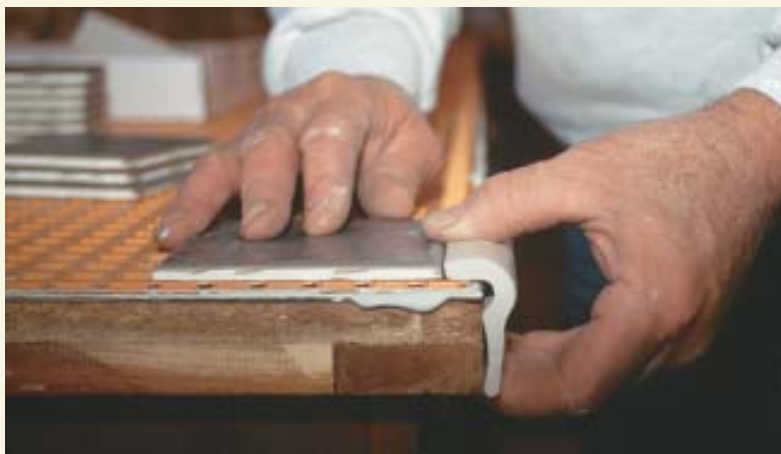
Figure 2. Precut sheets of textured polyethylene membrane go on over the cement (above left) and are bedded firmly in place with a wood float (above). An edge view of the proprietary membrane and dry-fitted pieces of tile and nosing reveals the undercut profile of the square depressions, which makes for a solid mechanical bond between the membrane and the layer of cement that will later accept the tile (left).
