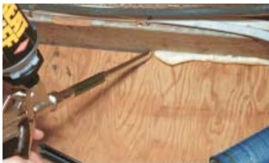
**With a slim nozzle and adjustable flow, a professional dispensing gun fits in tight spaces and minimizes the irritating blobs and bombs of foam common with straw-dispensed cans. The foam will keep for 30 days when left on the gun, but leaving it on longer could ruin the tool.**
