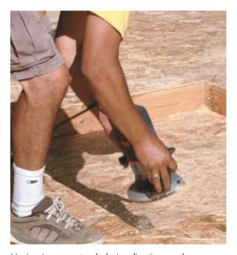
Moving in a counter-clockwise direction, work your way around the opening. The bearing guides the router for an accurate cut, and the whole process takes about a minute. Once you're done, you can nail off the sheathing and stand the wall.
