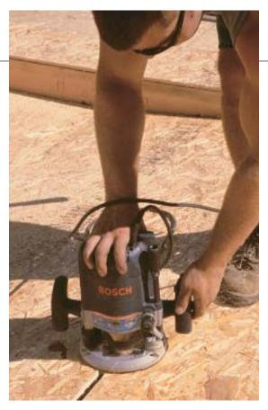
Cutting out door and window openings with a router saves time and makes a splinter-free cut. Start by making a hole with the claw end of your hammer. If you don't know exactly where the opening is, you can walk on the sheathing and feel where it flexes. Drop the bit through the hole, turn on the router, and move to the perimeter of the opening.
