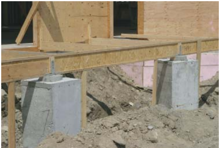
Figure 3. Engineered post anchors were tacked to spacer blocks on the I-joist grid (top). The anchors were set to within \frac{1}{8} inch before any concrete was poured. Circular nipple forms created a pier insert to help center the bottom of each column (above). The nipple was \frac{1}{2} inch smaller in diameter than the column interior to allow for leveling the base.
