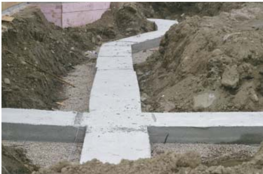
Figure 1. Rather than individual pads, a continuous footing permitted unlimited side-to-side adjustment for precisely placing the pier forms.
