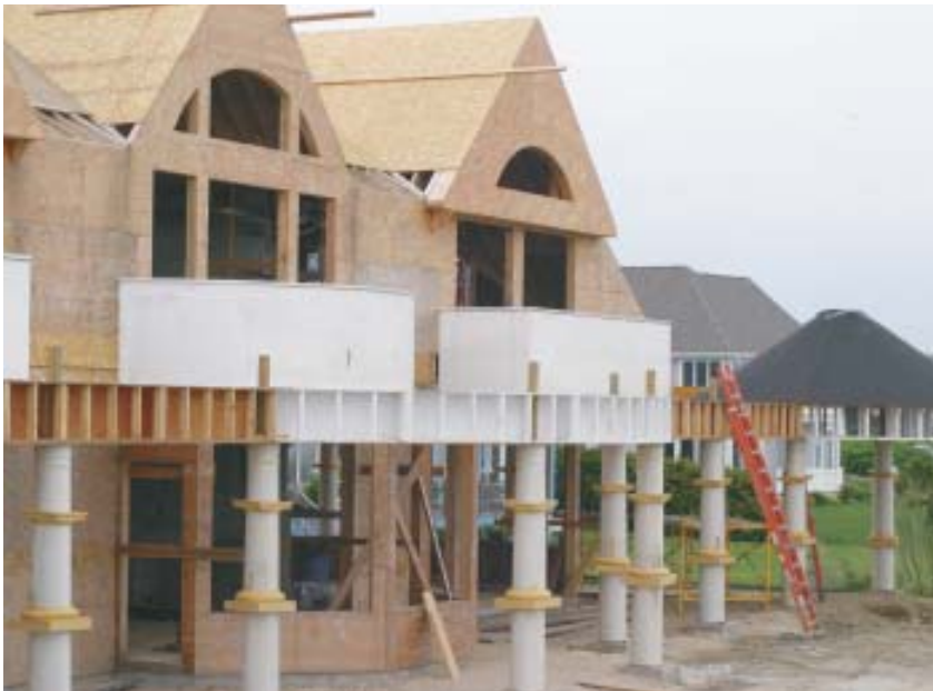
Figure 7. A nonstructural frame under the circular roof (top) aligns with the box beam entablature. The circular roof loads are carried to the columns by a site-laminated round top plate. Note how the plinth and capitals are wedged safely out of the way during construction (above).
