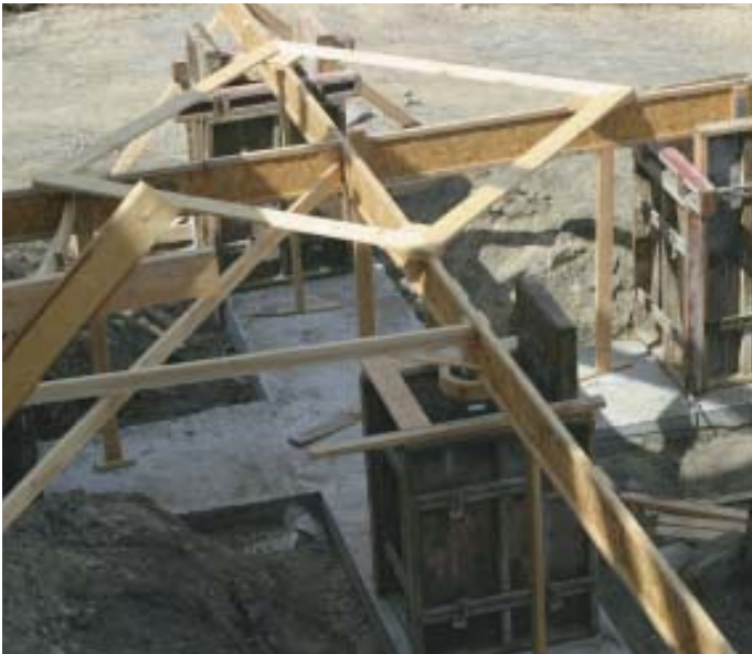
Figure 2. The author used I-joists instead of string for laying out the 17 porch columns, setting the bottom of the I-joists level with the top of the footings (left). This allowed the crew to accurately set the metal column anchors by tacking them to the I-joists. Spreaders, shimmed laser-straight off the building, set the center of the I-joist flange at the colonnade centerline. Two-by blocking tacked to both sides of the I-joist web at precise column locations established bull's-eye centers below which the pier forms could be set (right).
