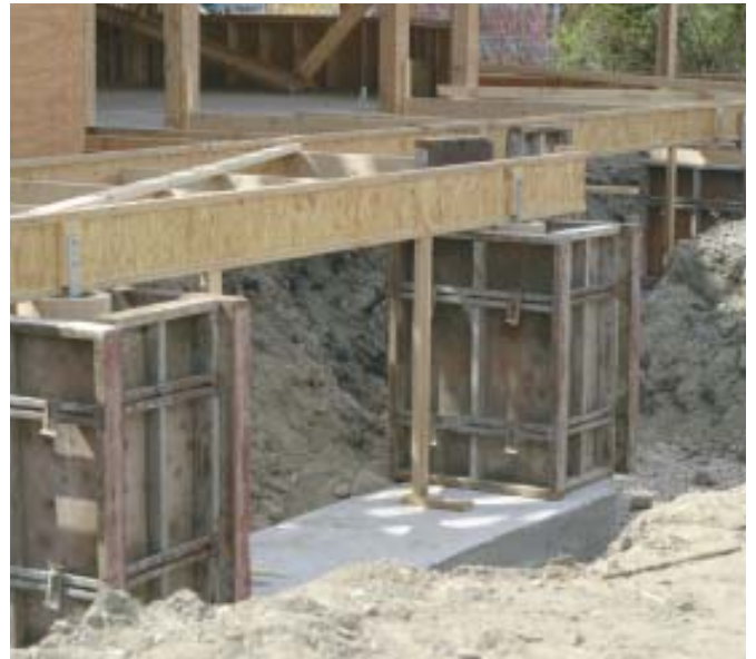
Figure 2. The author used I-joists instead of string for laying out the 17 porch columns, setting the bottom of the I-joists level with the top of the footings (left). This allowed the crew to accurately set the metal column anchors by tacking them to the I-joists. Spreaders, shimmed laser-straight off the building, set the center of the I-joist flange at the colonnade centerline. Two-by blocking tacked to both sides of the I-joist web at precise column locations established bull's-eye centers below which the pier forms could be set (right).
