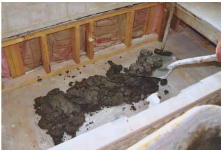
Figure 3. After tiling the tub platform, the author resets the tub in a bed of nonshrink grout (above). This supports the weight of the tub from the bottom rather than the lip. A layer of plastic or felt under the grout prevents the subfloor from absorbing moisture and swelling, which could lift the tub (right).
