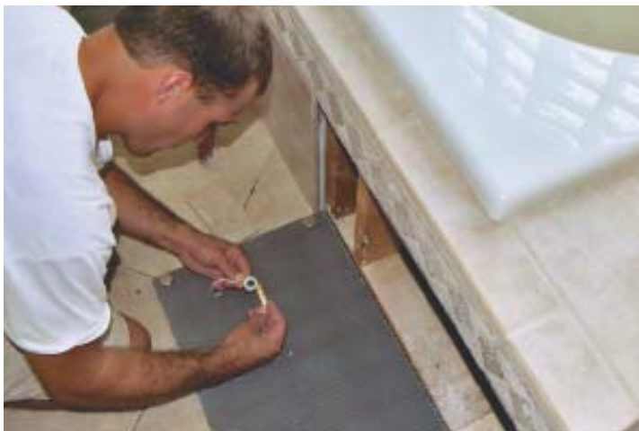
Figure 2. A nylon zip cord makes it easy to remove the access panel in the future. The cord is attached to a washer epoxied onto the back of the panel and is embedded in a bead of color-matching caulk around the panel's edge.
