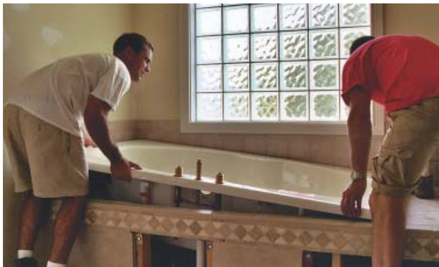
Figure 3. After tiling the tub platform, the author resets the tub in a bed of nonshrink grout (above). This supports the weight of the tub from the bottom rather than the lip. A layer of plastic or felt under the grout prevents the subfloor from absorbing moisture and swelling, which could lift the tub (right).
