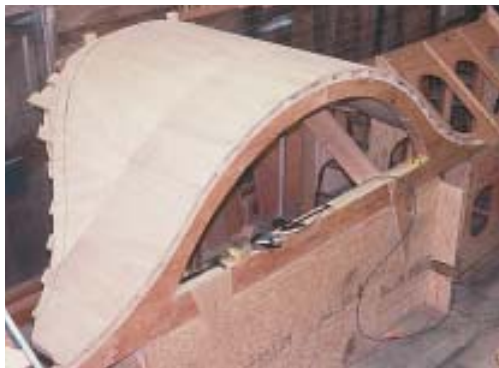
Plywood patterns, which were later installed as permanent structural bracing, served as straight-edge guides to establish the curved valley profile on the dormer.
