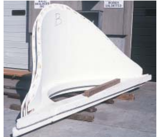
Foam-packed, primed, and stacked, the two dormers are ready for transport to the job site.
