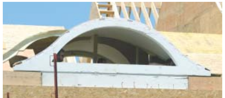
Roof panel sections and dormers were assembled in sequence, working end to end. The dormers’ weight is largely supported by the bearing walls directly below.
