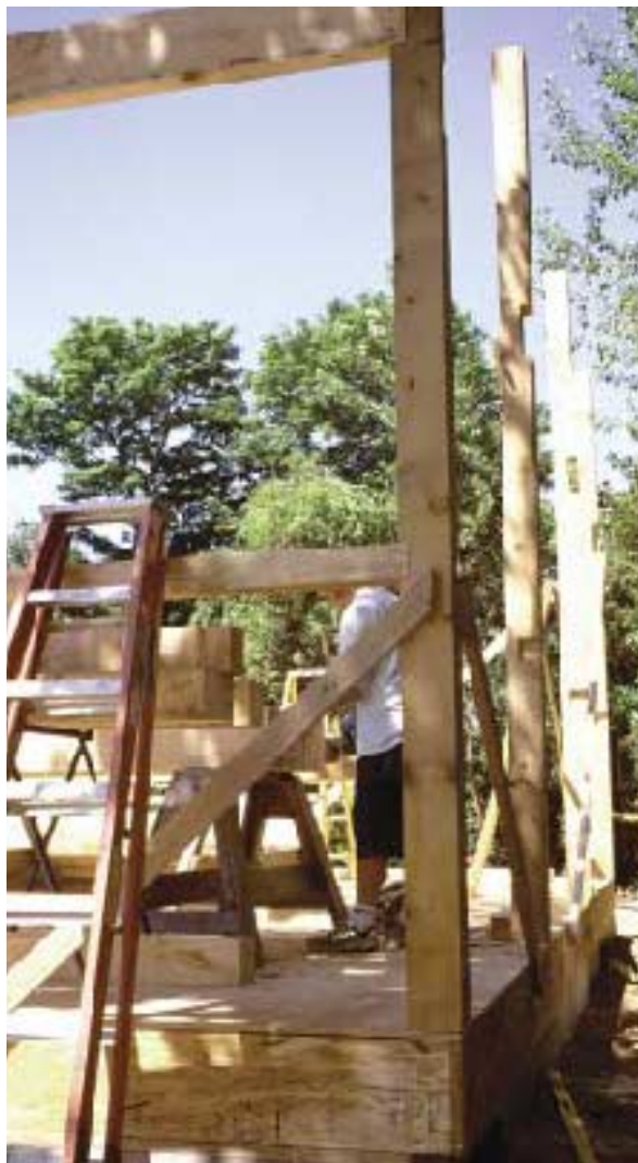
Figure 5. Posts are notched for a 2x10 ledger and 4x4 purlins before standing. This barn is being raised over a full foundation on an engineered-lumber deck frame. Pine floor boards will cover the plywood subfloor.
