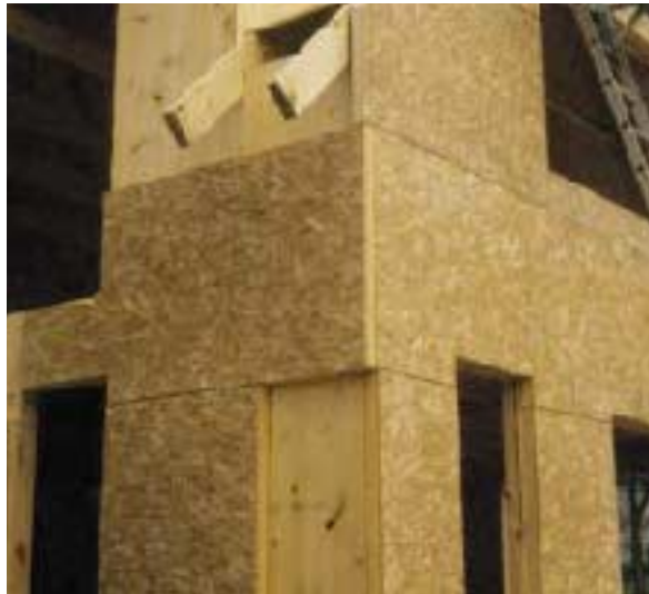
Figure 14. Exterior-mounted isocyanurate foam insulation panels with a laminated OSB nail-base facing provide moderate levels of insulation without altering the appearance of the interior walls and ceiling. Wall insulation is typically 1 inch thick, while roof cladding varies from 2 to 4 inches thick.
