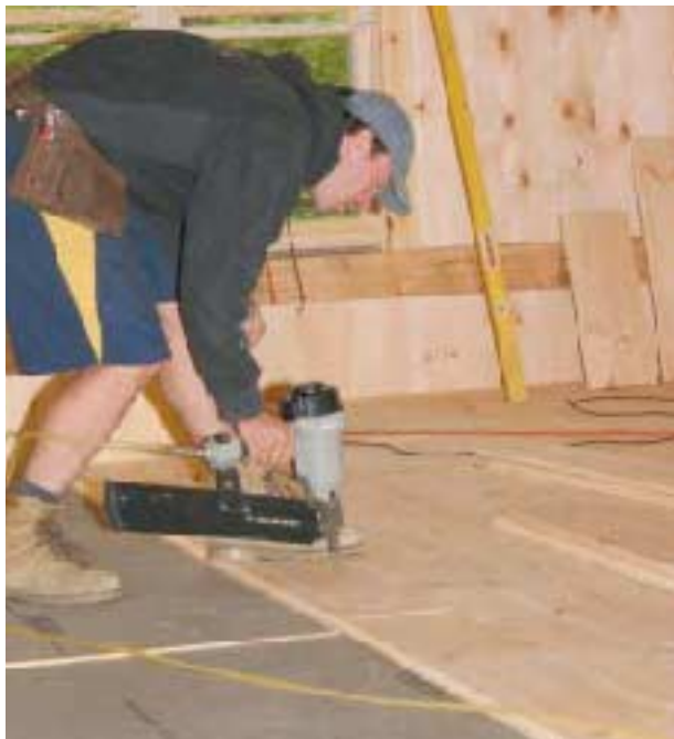
Figure 15. To insulate a wood-framed floor, the author sandwiches 1-inch-thick foam board with a fiber-reinforced facing between layers of 1x10 pine and nails the finish layer through to the framing.
