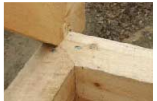
Figure 10. Mid-span posts are spiked with 12-inch-long galvanized nails, while end cuts and butt joints are nailed with lighter-gauge 10-inch nails (above). All holes get predrilled (left). Outside lintel corners are mitered with a 12-inch spike driven from the gable side (above right) to keep the joint tight (right).
