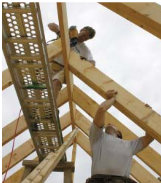
Figure 11. The rafters are carried by the hefty lintel and therefore don't have to align with the vertical framing below. Three-foot spacing is a nominal standard that can be adjusted to accommodate skylight openings and provide a balanced appearance.
