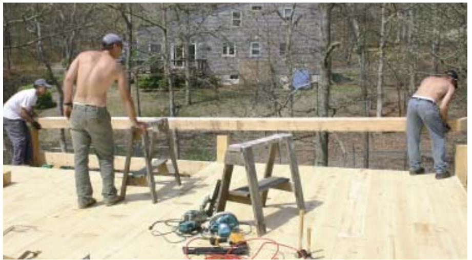
Figure 9. The posts are all cut to an equal height and are captured by notches in the lintel beam (above). The lintel is first scribed in place (left), then flipped over and kerfed with a circular saw set to cut 1 inch deep.
