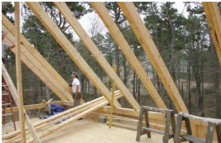
Figure 11. The rafters are carried by the hefty lintel and therefore don't have to align with the vertical framing below. Three-foot spacing is a nominal standard that can be adjusted to accommodate skylight openings and provide a balanced appearance.
