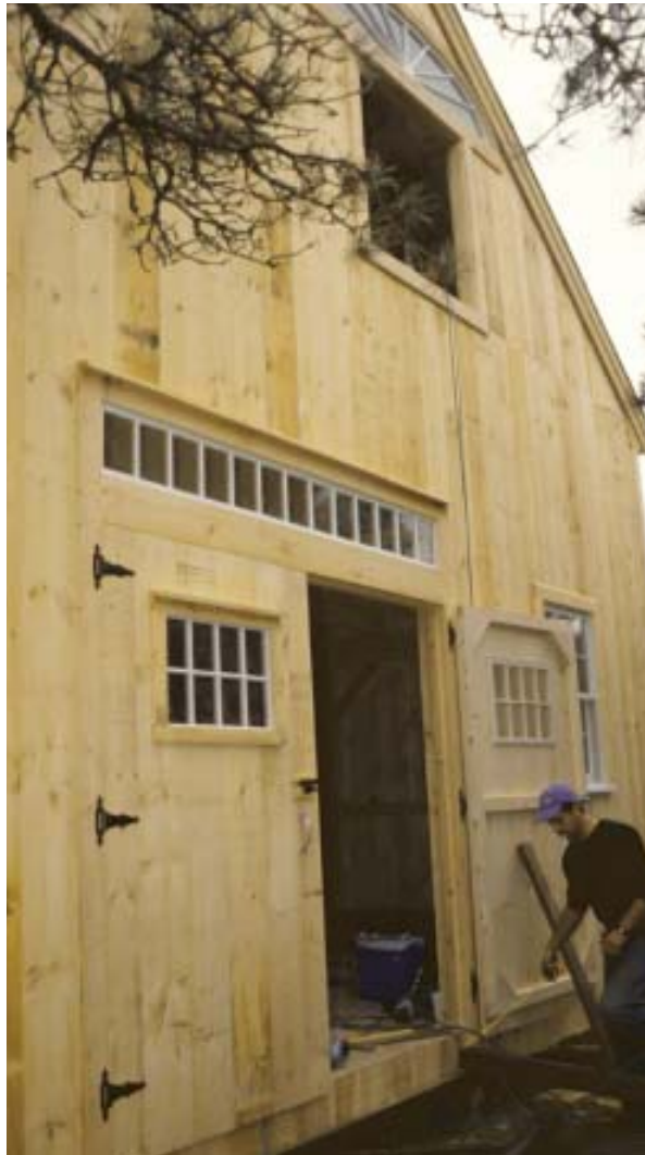
Figure 12. When shiplap pine sheathing does double duty as siding, the author uses urethane sealant behind door and window frames, and adds a sloped cap board to help drain water away. Deep roof overhangs also provide some protection on the eave sides.
