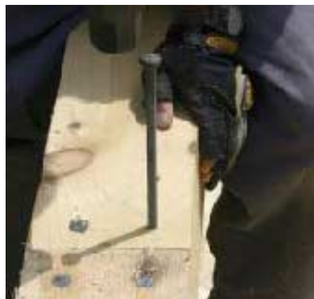
Figure 10. Mid-span posts are spiked with 12-inch-long galvanized nails, while end cuts and butt joints are nailed with lighter-gauge 10-inch nails (above). All holes get predrilled (left). Outside lintel corners are mitered with a 12-inch spike driven from the gable side (above right) to keep the joint tight (right).
