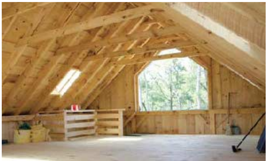
Figure 13. One-by-ten board sheathing installs quickly and provides a sturdy base for roofing. On an uninsulated roof, it's important to use 1-inch roofing nails in asphalt shingles to prevent unsightly penetrations on the interior ceiling.
