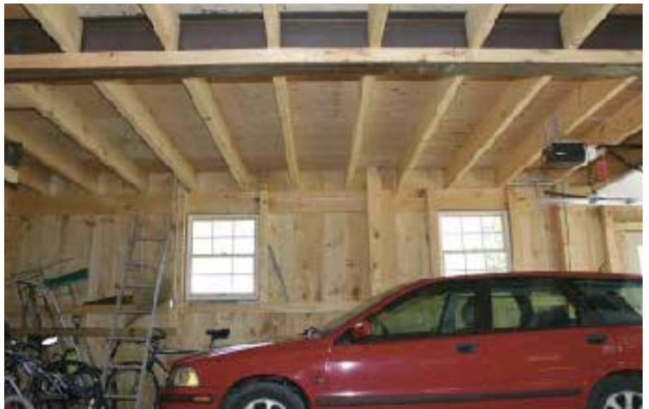
Figure 3. Engineered lumber and plywood find use in concealed locations, such as in a pine-veneered barn door header, or, in this case, in a subfloor that eventually will be concealed by a gypsum ceiling when the habitable space upstairs is finished.
