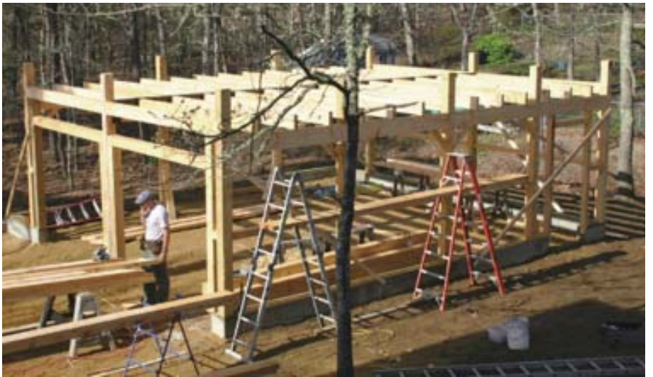
Figure 4. The second-floor joist ledger is notched into the outside face of the posts, which extend above the floor to create a knee-wall, adding headroom and storage space to the "loft." The posts are united with a continuous 6x6 lintel that carries the rafters.
