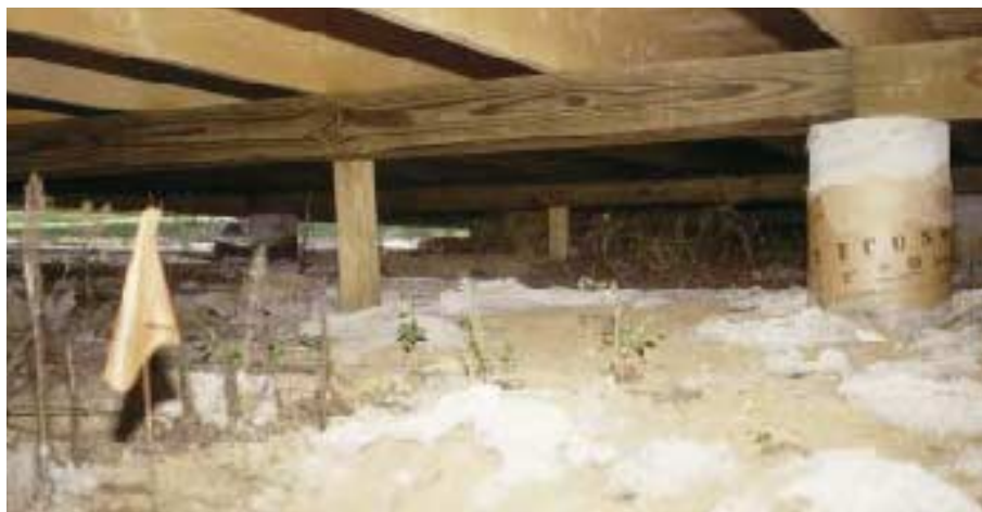
Figure 2. The author usually builds on a poured-concrete stem wall (above left). The slab area is filled and compacted, then poured later. Although a building inspector may occasionally require post anchors to tie the vertical structural members to the foundation, toe-nailed posts are generally accepted, provided the mudsill is properly bolted (above). Another option is concrete piers and pressure-treated carriage beams, which greatly reduce excavation and foundation costs (left).
