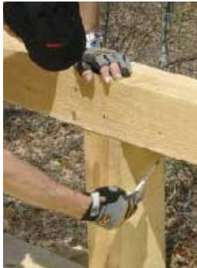
Figure 9. The posts are all cut to an equal height and are captured by notches in the lintel beam (above). The lintel is first scribed in place (left), then flipped over and kerfed with a circular saw set to cut 1 inch deep.
