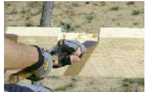
Figure 9. The posts are all cut to an equal height and are captured by notches in the lintel beam (above). The lintel is first scribed in place (left), then flipped over and kerfed with a circular saw set to cut 1 inch deep.
