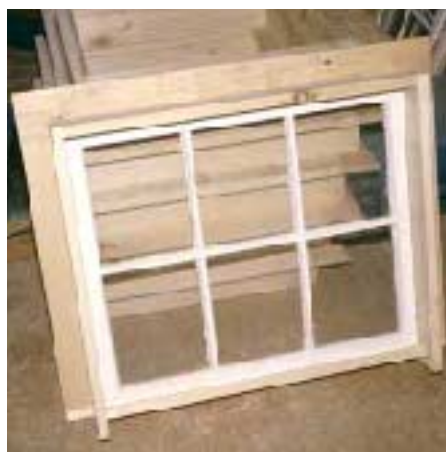
Figure 6. As a touch of authenticity, the author often uses recycled wood window sash and installs them in site-made pine frames.
