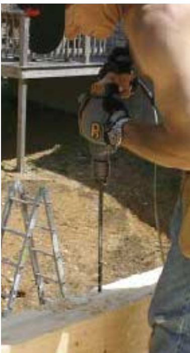
Figure 10. Mid-span posts are spiked with 12-inch-long galvanized nails, while end cuts and butt joints are nailed with lighter-gauge 10-inch nails (above). All holes get predrilled (left). Outside lintel corners are mitered with a 12-inch spike driven from the gable side (above right) to keep the joint tight (right).
