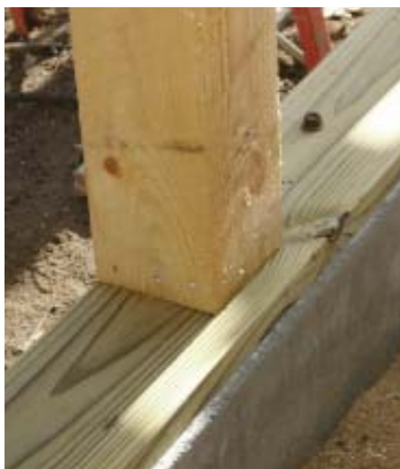
Figure 2. The author usually builds on a poured-concrete stem wall (above left). The slab area is filled and compacted, then poured later. Although a building inspector may occasionally require post anchors to tie the vertical structural members to the foundation, toe-nailed posts are generally accepted, provided the mudsill is properly bolted (above). Another option is concrete piers and pressure-treated carriage beams, which greatly reduce excavation and foundation costs (left).
