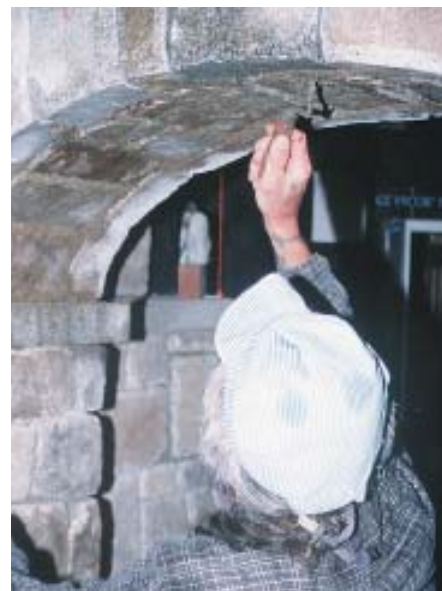
Figure 4. The underside, or soffit, is laid between the ring stones. Mortar and masonry rubble fill the void behind the face stones. As he places each stone, the author spreads sand on the form and packs a layer into the joints before the mortar (left and below left). The sand helps keep the finished face clean and falls out when the form is pulled, leaving recessed joints. Only minor pointing is needed to finish (below).
