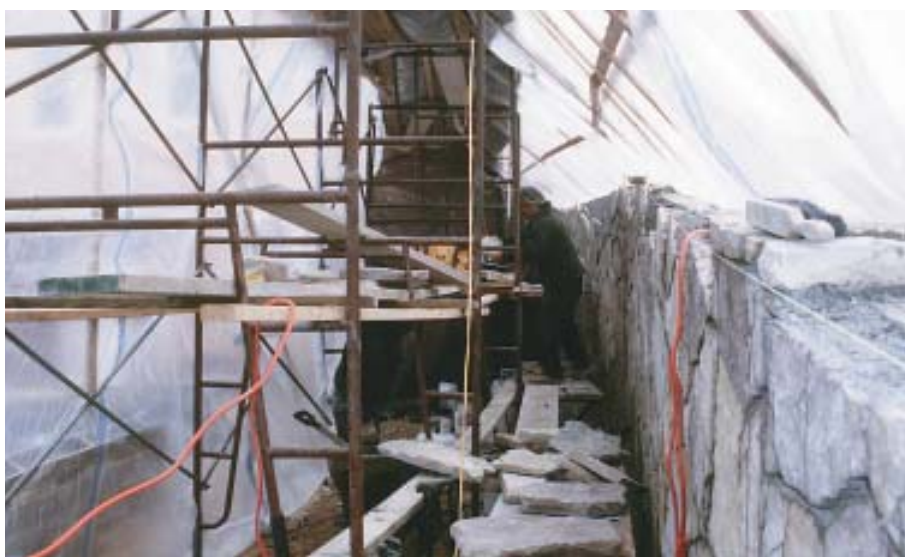
Figure 9. The crew constructs a temporary shelter of pipe scaffold, lumber, and poly sheeting over the primary work area. Propane-fired heaters keep the materials and masons above the freezing mark in cold weather.
