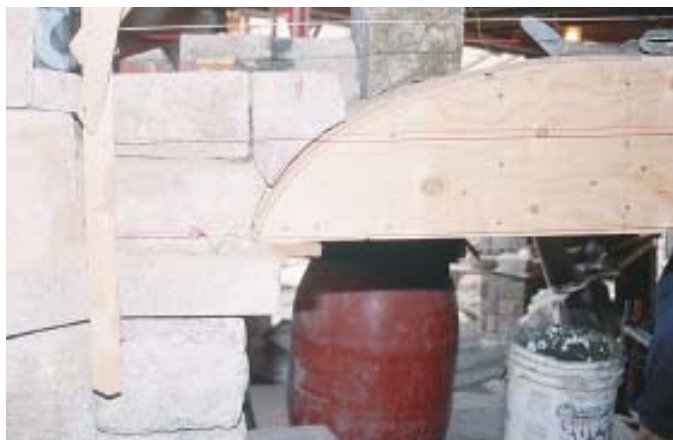
Figure 3. Wood shims under the arch form ensure easy removal later. The author relies on the builder to construct the form.
