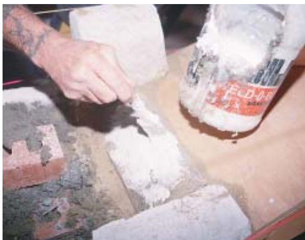
Figure 5. Although Portland cement forms a naturally strong bond with stone, the author brushes all mating surfaces with an acrylic binder to improve adhesion.
