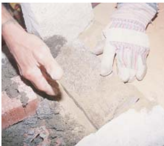
Figure 4. The underside, or soffit, is laid between the ring stones. Mortar and masonry rubble fill the void behind the face stones. As he places each stone, the author spreads sand on the form and packs a layer into the joints before the mortar (left and below left). The sand helps keep the finished face clean and falls out when the form is pulled, leaving recessed joints. Only minor pointing is needed to finish (below).
