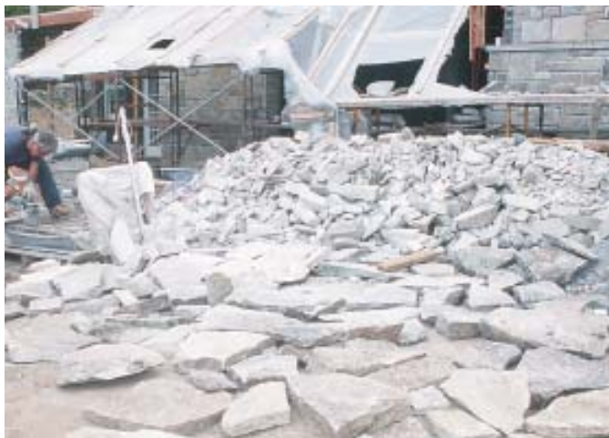
Figure 2. An ashlar pattern requires each stone to have straight, man-made edges and be laid in a close-fitting, angular design. The waste factor runs as high as 40%, producing a considerable pile of rubble as the work progresses.
