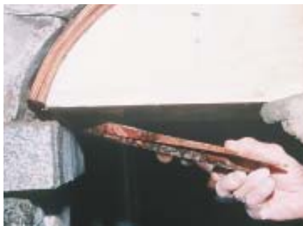
Figure 3. Wood shims under the arch form ensure easy removal later. The author relies on the builder to construct the form.
