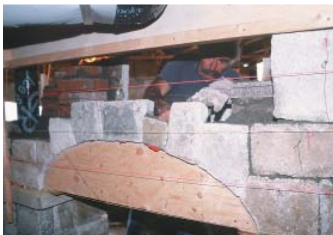
Figure 6. Mortar is slippery when wet. Shims and wire twists stabilize individual stones until the cement hardens.
