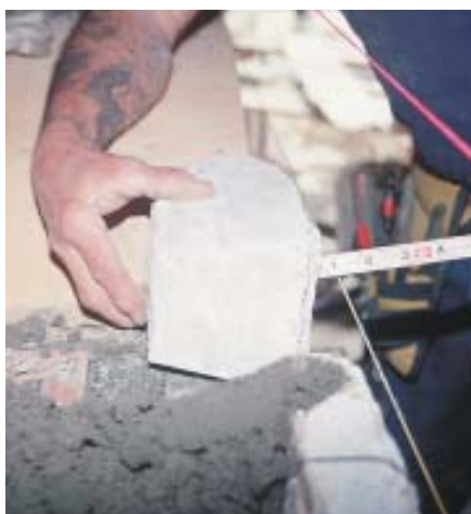
Figure 6. Mortar is slippery when wet. Shims and wire twists stabilize individual stones until the cement hardens.
