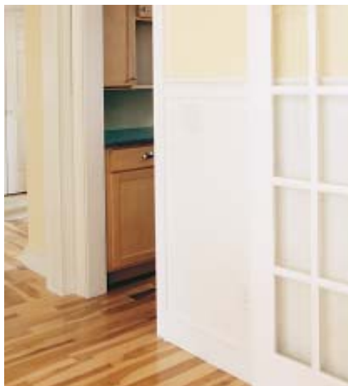
Figure 3. Using MDF wainscoting in a variety of heights complements standard stool and head casing heights, creating a much livelier interior. The author installs the wainscot with construction adhesive and a few 18-gauge brads to hold it in position while the glue sets — making for fewer nail holes to fill. Windsor casing, rabbeted on the bottom, makes a good cap (far right).
