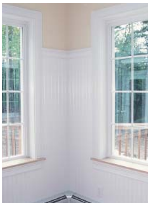
Figure 3. Using MDF wainscoting in a variety of heights complements standard stool and head casing heights, creating a much livelier interior. The author installs the wainscot with construction adhesive and a few 18-gauge brads to hold it in position while the glue sets — making for fewer nail holes to fill. Windsor casing, rabbeted on the bottom, makes a good cap (far right).
