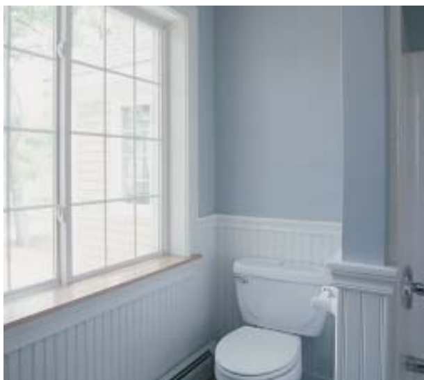
Figure 3. Using MDF wainscoting in a variety of heights complements standard stool and head casing heights, creating a much livelier interior. The author installs the wainscot with construction adhesive and a few 18-gauge brads to hold it in position while the glue sets — making for fewer nail holes to fill. Windsor casing, rabbeted on the bottom, makes a good cap (far right).
