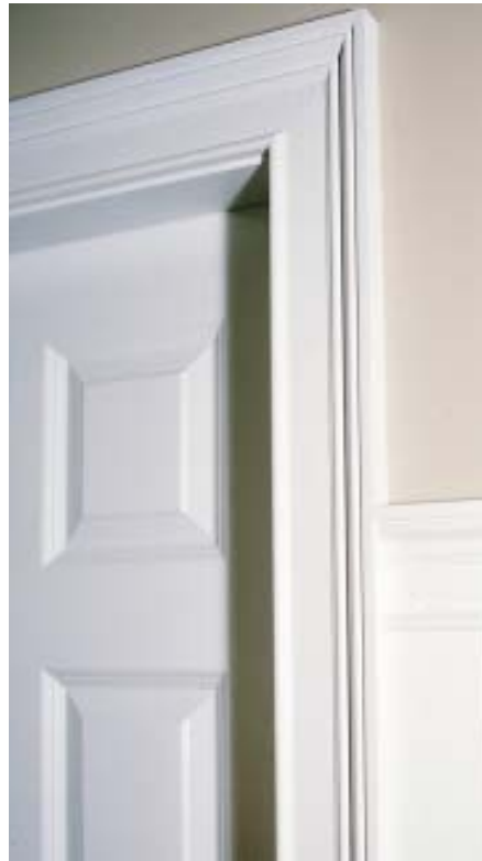
Figure 2. Windsor casing made from MDF costs about half what the same profile costs in wood. But because it's more dimensionally stable than wood, MDF miters don't open with seasonal moisture changes. The author uses a fast-setting adhesive to guarantee tight joints.
