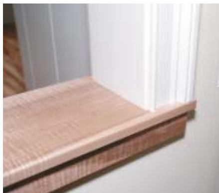
Figure 1. Using MDF for most of the trim leaves room in the author's budget to use attractive figured hardwoods in high-visibility areas like sills, window seats, and other built-ins.
