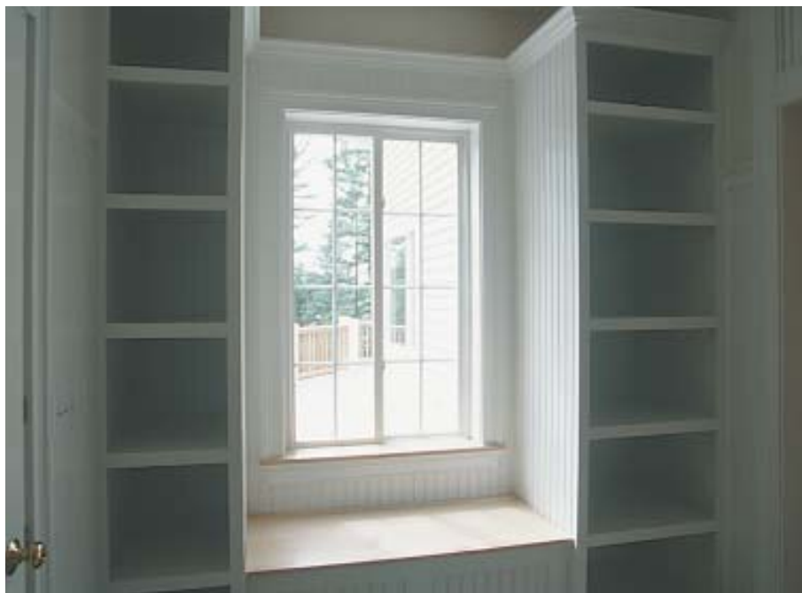
Figure 1. Using MDF for most of the trim leaves room in the author's budget to use attractive figured hardwoods in high-visibility areas like sills, window seats, and other built-ins.
