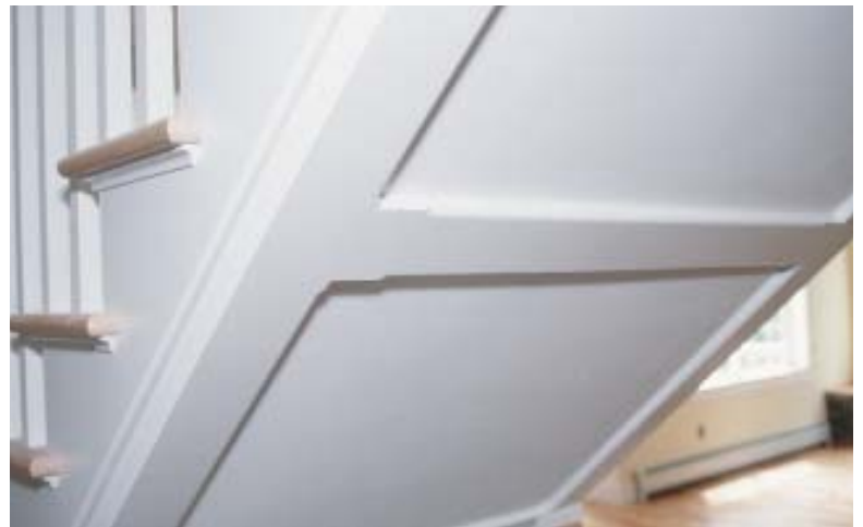
Figure 2. Windsor casing made from MDF costs about half what the same profile costs in wood. But because it's more dimensionally stable than wood, MDF miters don't open with seasonal moisture changes. The author uses a fast-setting adhesive to guarantee tight joints.
