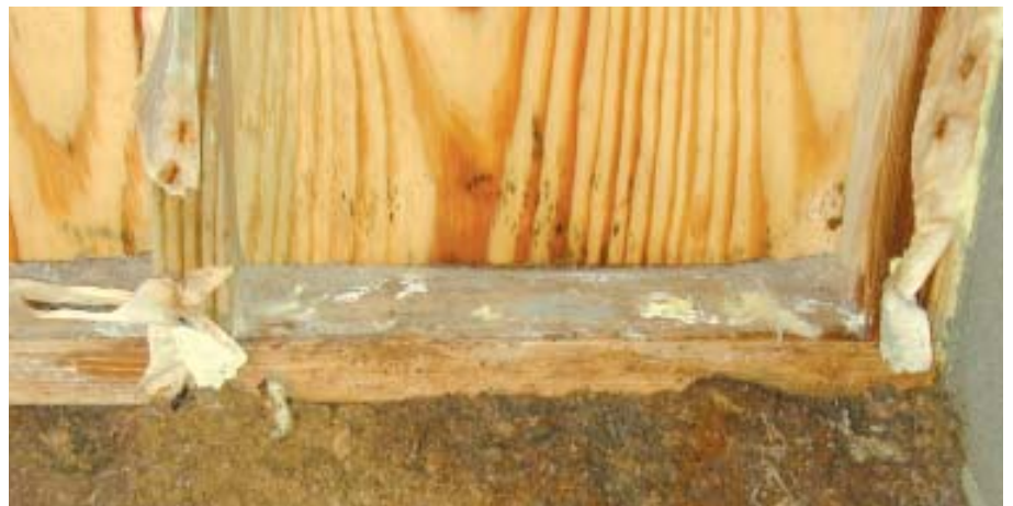
Figure 3. Moisture condensing on the cold masonry columns (top) on the perimeter of the crawlspace was wicking into the adjacent cripple wall framing and insulation batts. There was fungus even on the surface of the treated wood wall plate (above).
