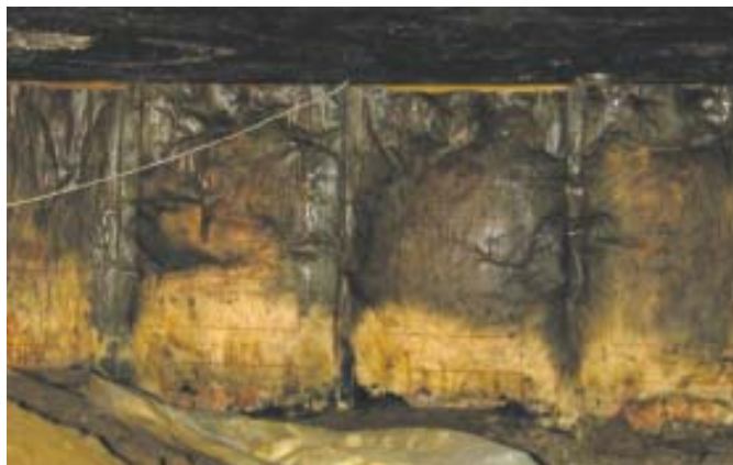
Figure 4. In the worst parts of the crawlspace, wood and insulation facings were covered with slick black coatings of wet, slimy mold (right and below). The presence of mole crickets (bottom) also indicated that the space was constantly damp.
