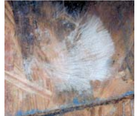
Figure 2. Every surface in the crawlspace was dripping wet, including electrical outlets (left). Even the staples holding insulation batts in place were rusty and gleaming with moisture (below left). Droplets of water were also visible on the filaments of this white fungus (below).
