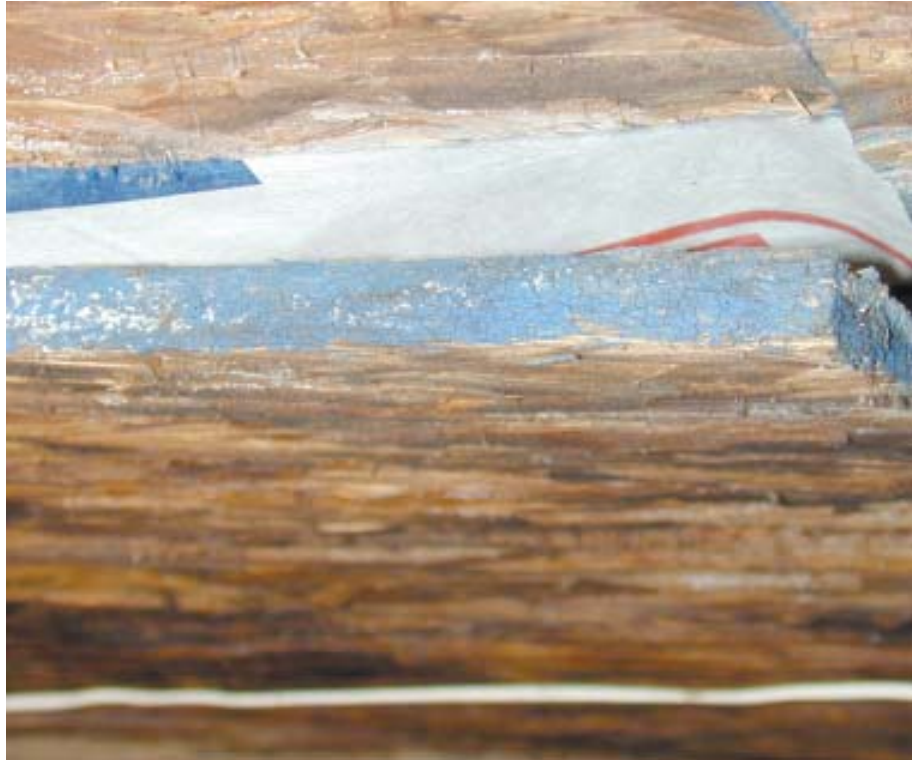
Figure 6. OSB and Tyvek between the crawlspace and the floor protected the floor structure from damage, saving the floor (and perhaps the house) from total ruin. The OSB was heavily attacked by fungus, but could still be cleaned up with brushes and a borate solution.
