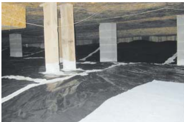
Figure 8. To finish off the space, the author's crew seals the vent openings with duct tape and mastic (top left), and applies a poly ground cover, sealed to the base of the crawlspace wall (top right). Carpeting protects the 6-mil poly (above) in the area near the access, creating the perception of a space that should be treated with care.
