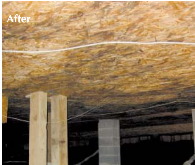
Figure 1. Upon opening the crawlspace door, the author saw large, obvious patches of white wood rot and black mold (right and below). The OSB ceiling looks considerably better at the end of the job (bottom), after the crew has scrubbed it with a borate solution.
