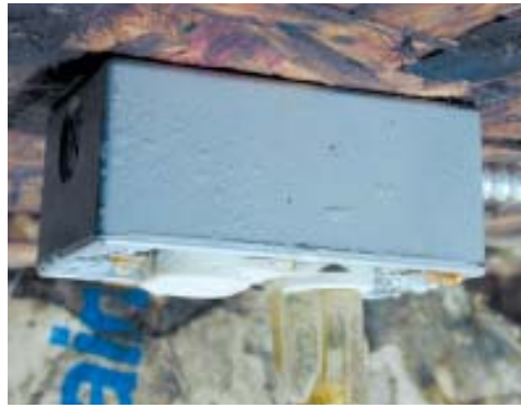
Figure 2. Every surface in the crawlspace was dripping wet, including electrical outlets (left). Even the staples holding insulation batts in place were rusty and gleaming with moisture (below left). Droplets of water were also visible on the filaments of this white fungus (below).
