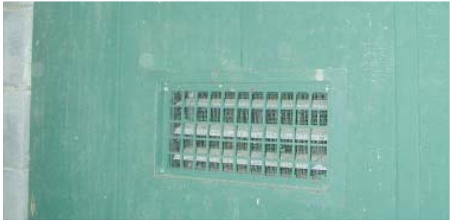
Figure 5. The entire crawlspace was equipped with just two small vents. One is shown here as viewed from outside the crawlspace under the exterior deck.
