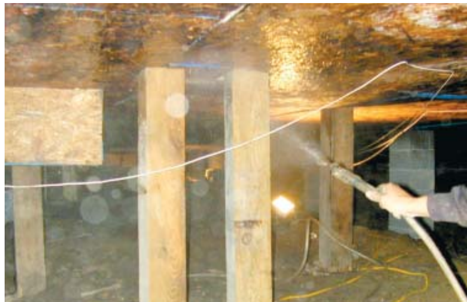
Figure 7. The author's old battery-powered sprayer (top) is small enough to drag into hard-to-access spaces, and allows him to saturate the underfloor OSB with a solution of Tim-bor borate, killing mold, rot organisms, and insects without toxic risk to people (above).
