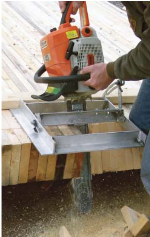
Figure 4. A chainsaw has enough depth of cut to cut heads and tails in a single pass. This saw is attached to a custom-made shoe; an off-the-shelf model is available from Big Foot Tools.
