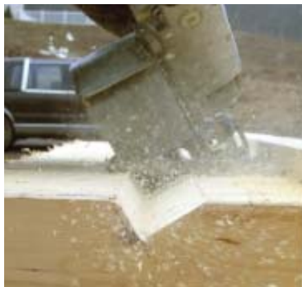
Figure 6. Here, the author uses a custom-made dado saw to hog out birdsmouths in a single pass.
