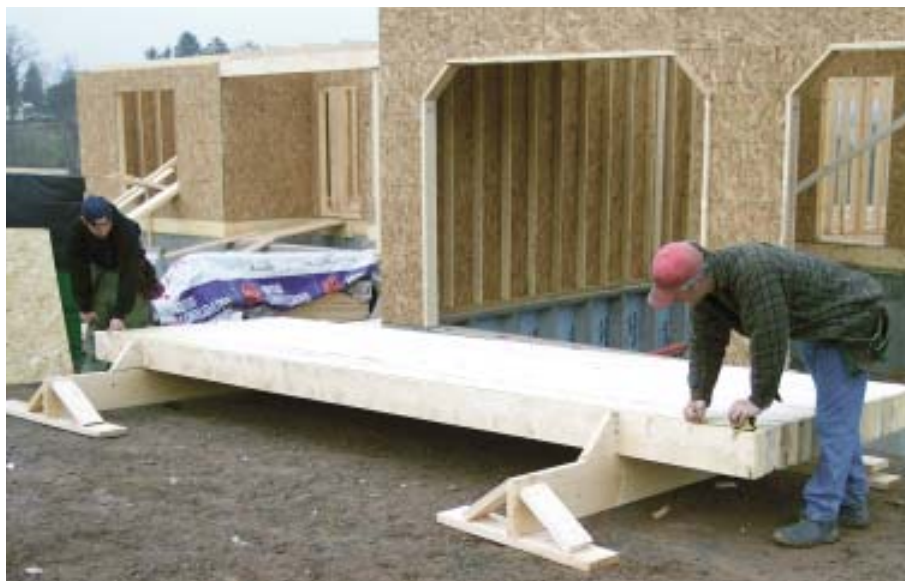
Figure 1. The rafters are supported by a pair of simple racks and are kept upright by the triangular blocks at the ends.
