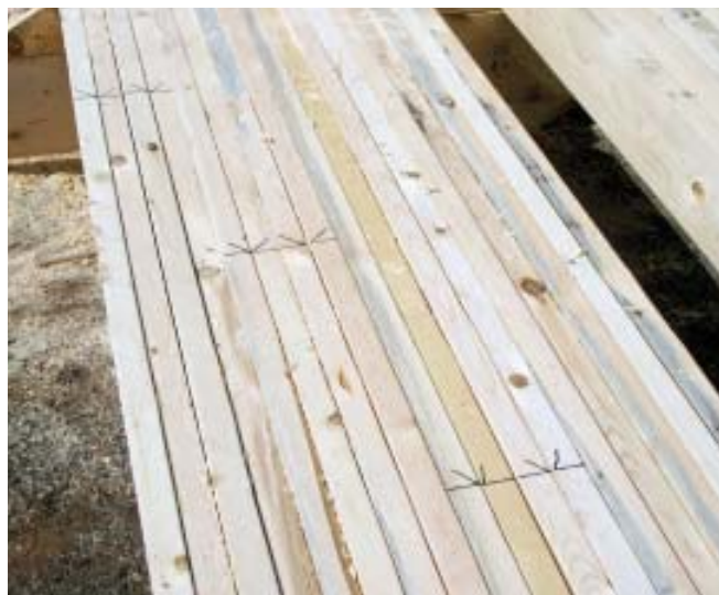
Figure 8. Hip jacks are laid out in pairs, lefts and rights (left). In the photo at right, the three shortest pairs for two hips have been marked. The offcuts will be long enough to produce the next three pairs.
