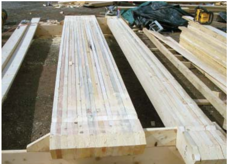
Figure 3. Twelve-inch spacer blocks separate groups of rafters on the racks so that different cuts can be made, increasing the efficiency of both the stacking and cutting operations.
