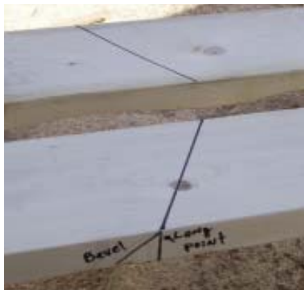
Figure 9. The bevel is ready to be cut on this pair of hip jacks. The birdsmouths have already been cut on the other end.
