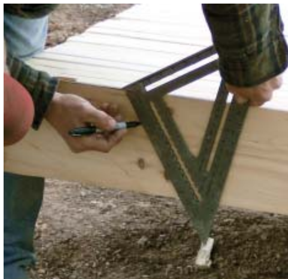
Figure 2. Layout is done on the outer pieces (right), and a chalk line is used to transfer the cut lines to the pieces in between (below).
