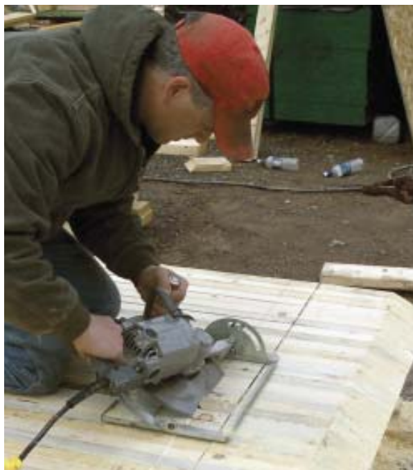
Figure 5. A swing-table saw makes possible the steep angles required for birdsmouths. Here, the birdsmouths on 50 rafters are made with just two long cuts.
