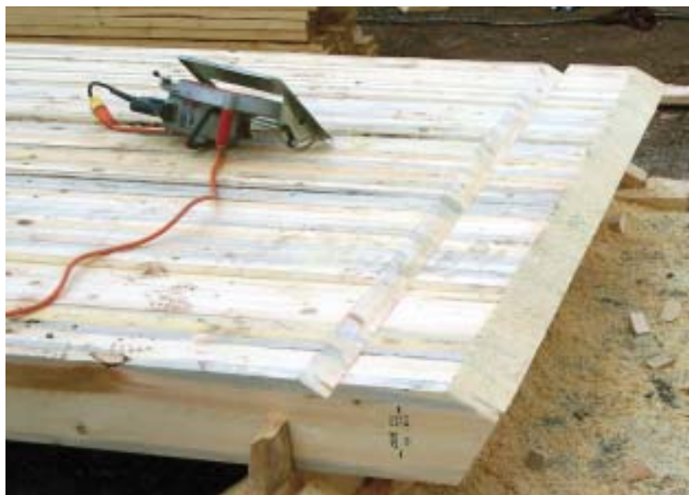
Figure 5. A swing-table saw makes possible the steep angles required for birdsmouths. Here, the birdsmouths on 50 rafters are made with just two long cuts.
