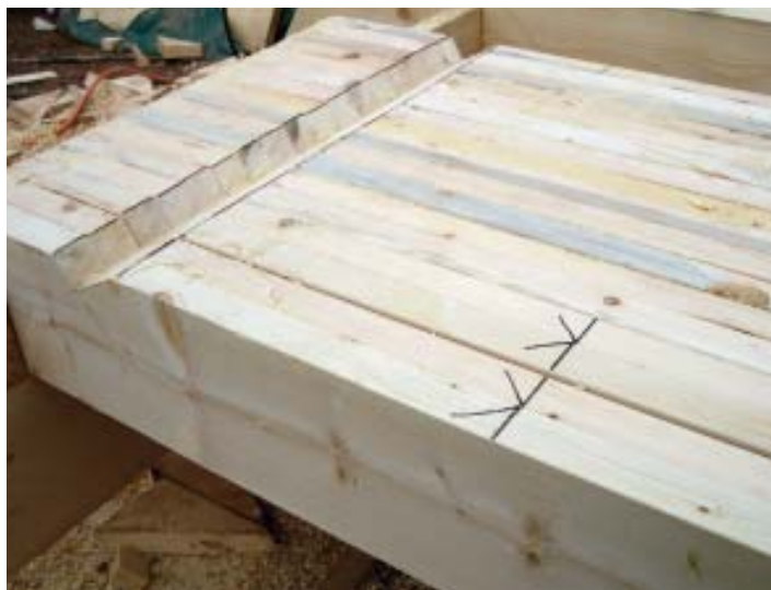
Figure 8. Hip jacks are laid out in pairs, lefts and rights (left). In the photo at right, the three shortest pairs for two hips have been marked. The offcuts will be long enough to produce the next three pairs.
