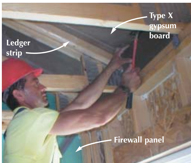
Figure 5. Where the area separation wall meets the roof, sheets of 5/8-inch type X gypsum board protect the underside of the roof sheathing in the two adjoining rafter bays on each side.
