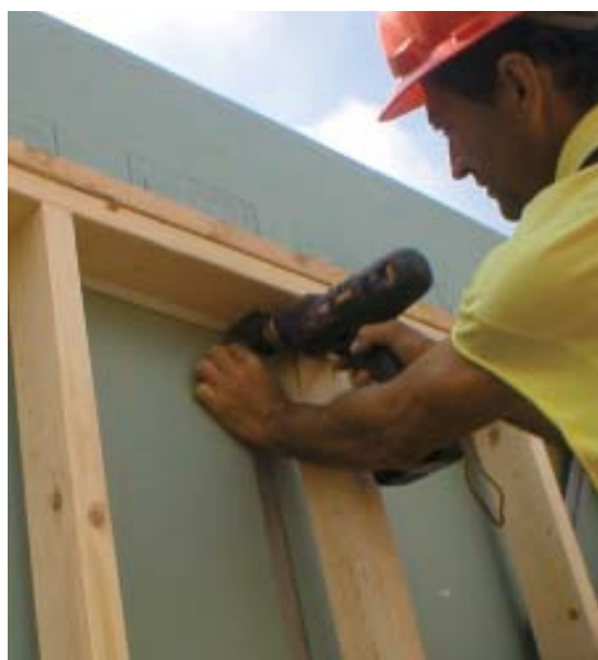
Figure 4. The double layer of gypsum board at the center of the area separation wall assembly is fastened to the adjacent framing with aluminum “breakaway clips.” In the heat of a fire, the clips soften and melt, allowing the burning unit to collapse without pulling down the firewall or the neighboring unit on the other side.
