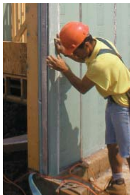
Figure 6. A carpenter installs a strip of fire-blocking to close the gap where a short section of exterior garage wall will butt against the area separation wall.
