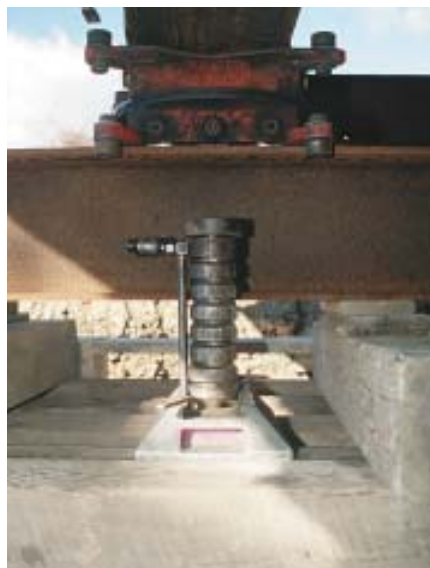
Figure 7. Four-foot lengths of 6x7-inch timbers are stacked to support the main steel H-beams. To ensure stability, the cribbing must be shimmed or shoveled dead level (above). One layer is blocked solid to support the jack (right). The unified jacking system manifold also provides an instant readout on the weight each jack lifts (below).
