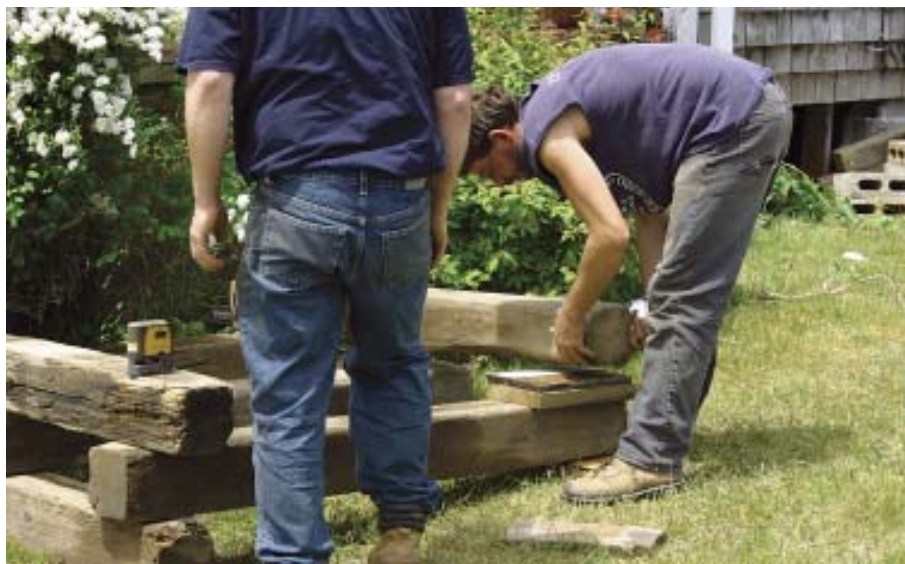
Figure 7. Four-foot lengths of 6x7-inch timbers are stacked to support the main steel H-beams. To ensure stability, the cribbing must be shimmed or shoveled dead level (above). One layer is blocked solid to support the jack (right). The unified jacking system manifold also provides an instant readout on the weight each jack lifts (below).
