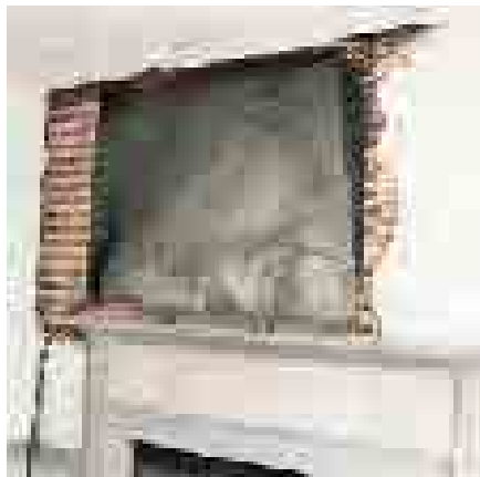
Figure 2. A parge-coat of masonry cement held the bricks steady for lifting and transportation (above). Restoration efforts included making a temporary access hole (shown patched in the photo at right) to send a small mason inside the chimney to repair and reline the three throats and flues.
