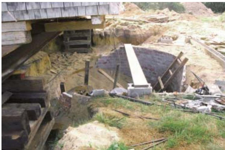
Figure 1. The house originally stood only inches above grade on a low brick perimeter, with intermediate wood posts at key framing junctions in the floor system. With the exception of a circular root cellar under the ell (above), there was virtually no clearance below the joists. In spite of this, the wood was in remarkably good condition (right).
