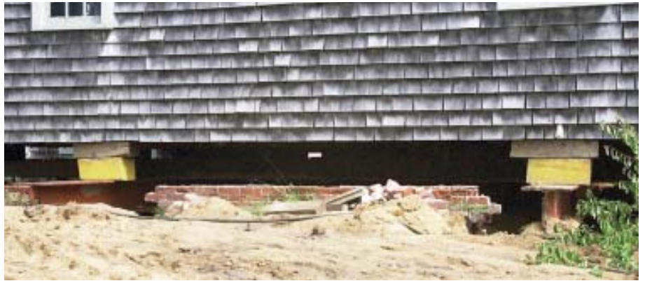
Figure 5. After carefully removing every other stone supporting the three chimneys and pouring a unifying reinforced concrete slab between them, the author slipped two needle beams beneath the masonry, initially jacking them just enough to transfer the load.
