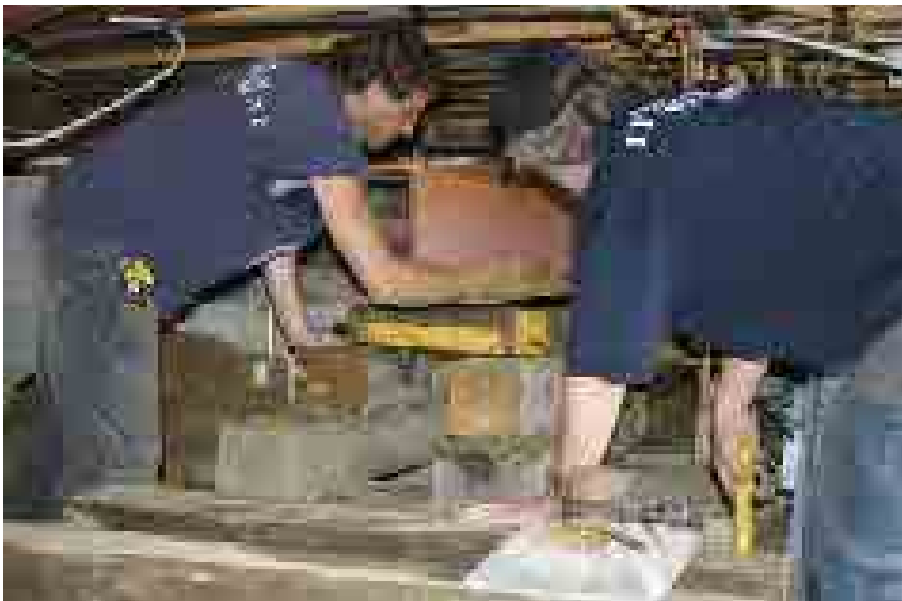
Figure 6. Rollers facilitate beam placement under the structure. The beam is chained to the backhoe bucket to keep it from launching itself forward like a battering ram.
