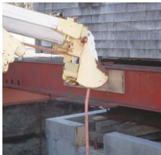
Figure 8. Two-way Hevi-Haul skates (top), are used to roll a building on or off the foundation as well as for alignment above a new foundation before lowering the house into place. Here, the house is winched forward on one axis (above) and nudged into position with a derrick arm on the other axis (left).
