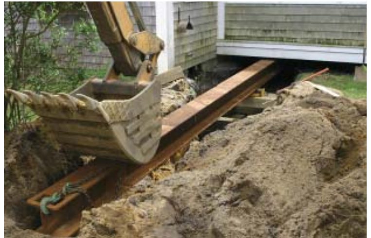
Figure 6. Rollers facilitate beam placement under the structure. The beam is chained to the backhoe bucket to keep it from launching itself forward like a battering ram.
