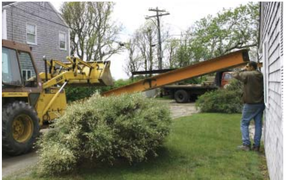
Figure 3. While the author swings a two-ton main beam into position with the backhoe, a worker makes sure the far end doesn't take out the neighbors' place across the street.
