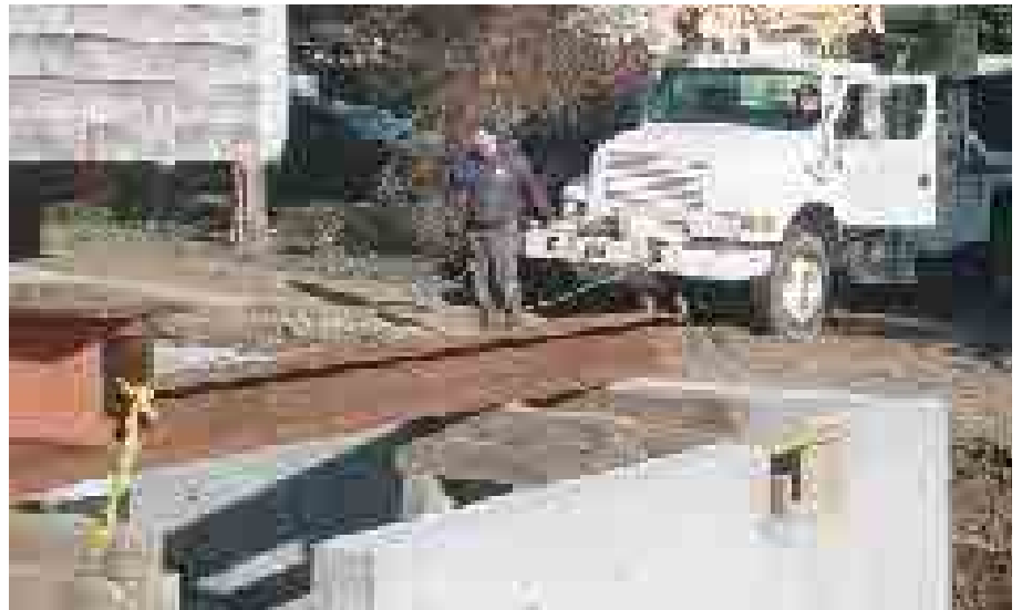
Figure 8. Two-way Hevi-Haul skates (top), are used to roll a building on or off the foundation as well as for alignment above a new foundation before lowering the house into place. Here, the house is winched forward on one axis (above) and nudged into position with a derrick arm on the other axis (left).
