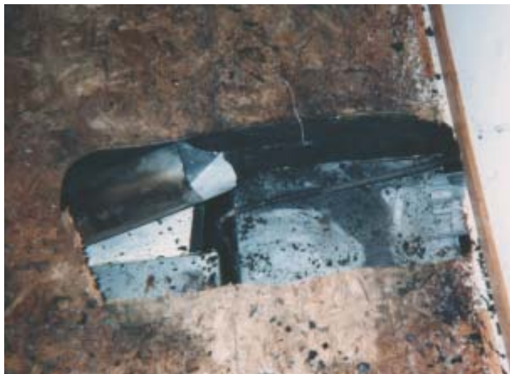
A fire was ignited in this crawlspace by a lightning strike that arced from the flexible gas tubing to a metal heating duct. The local fire department arrived in time to save the structure.
